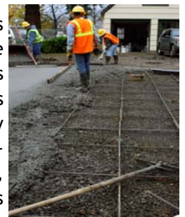
Dale Woodin Concrete
