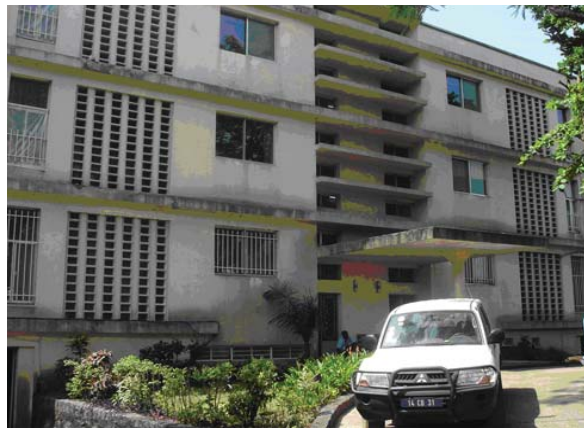
Exterior of Signal Hill embassy housing
