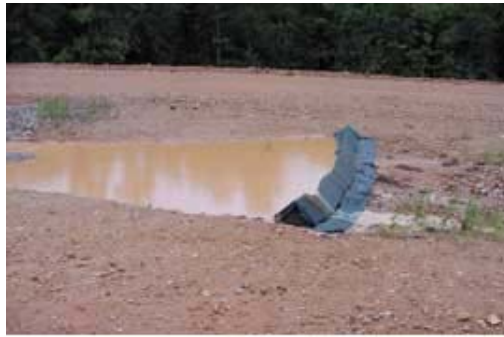
Geotextile Triangular Dike
