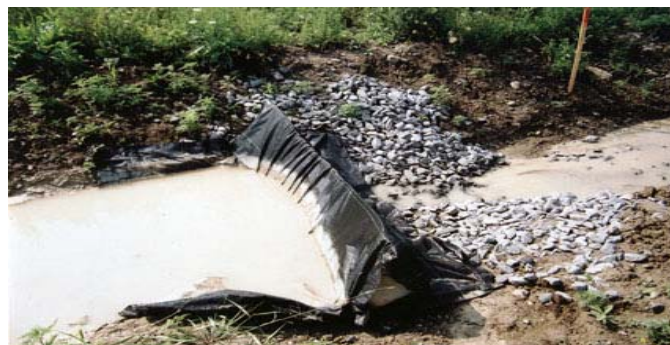
Geotextile Triangular Dike with Rock Backing
