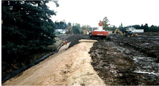
Retention Blanket in Ditch
