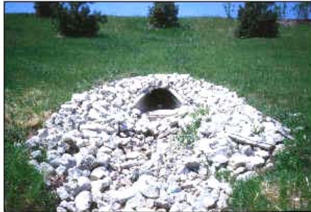
Riprap at Culvert Outlet
