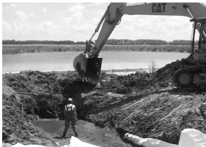
Centerline pipe on ND 1.
