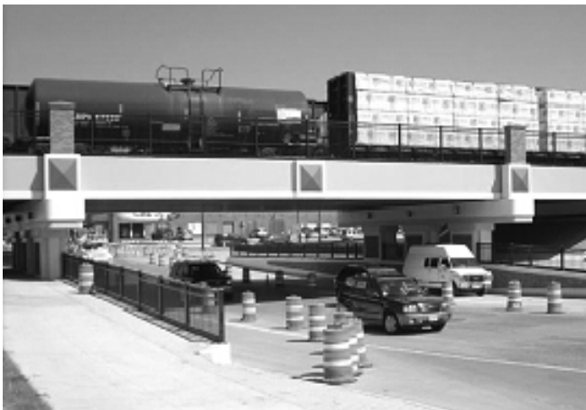
Railroad underpass on University Drive, Fargo.
