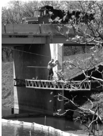
Worker cuts off pier face on Apple Creek Bridge, ND 1804.
