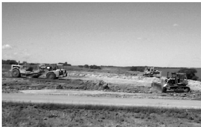
Widening roadway on ND 200.
