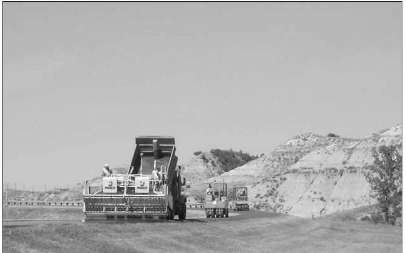
Maintenance workers place a sealcoat on a roadway.
