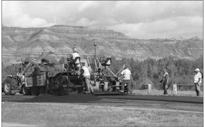
Asphalt paving work in the badlands near the US 85 corridor.
