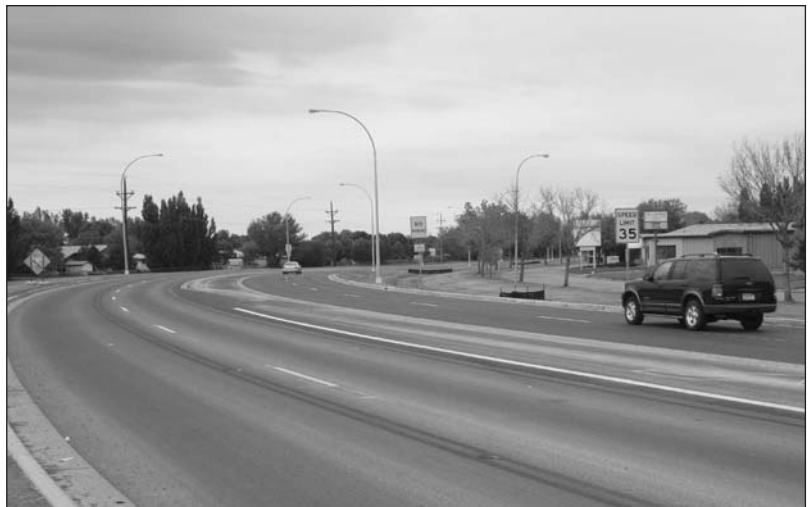
Traffic flow was greatly improved on Airport Road.
