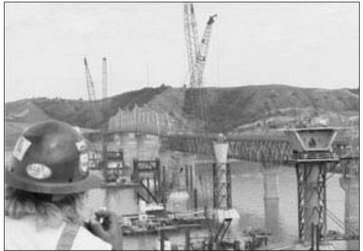
Construction activities on the Four Bears Bridge.
