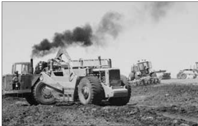
About 3.5 million cubic yards of earth were moved on US 2.
