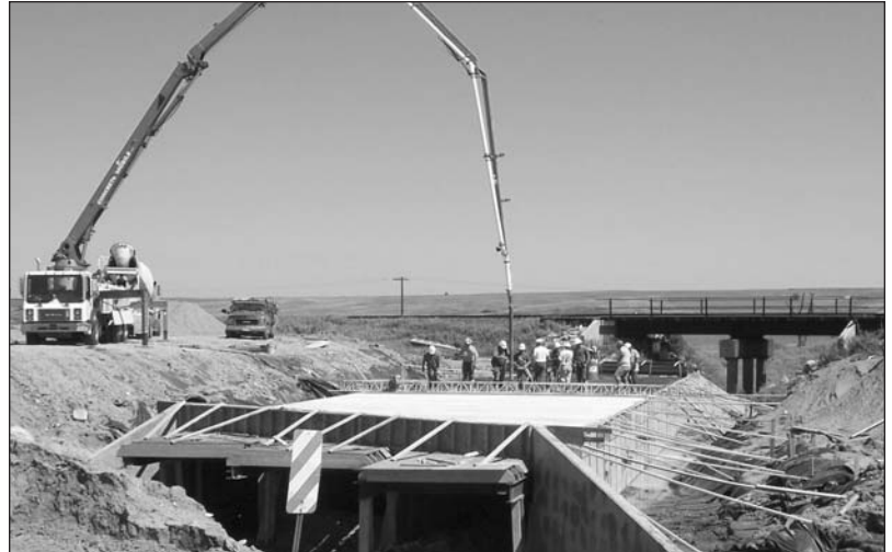
Concrete placement for a structure on the US 52 project.
