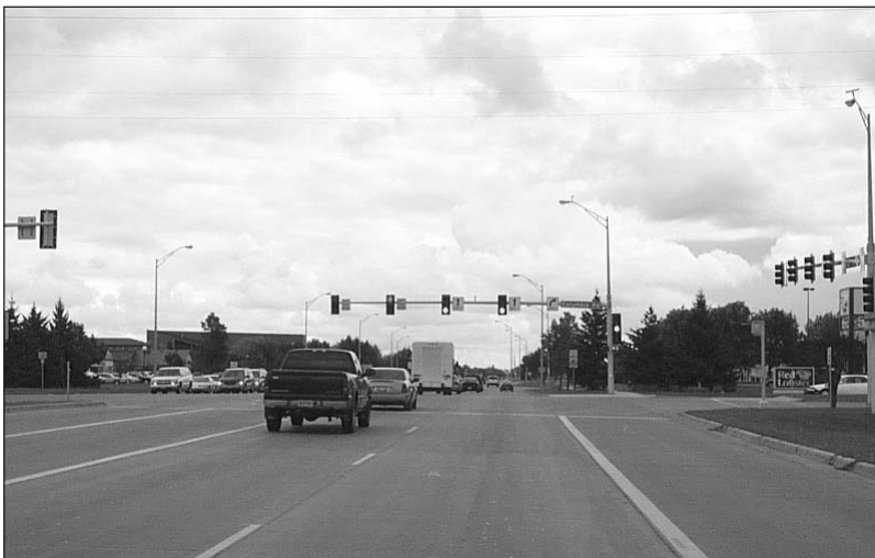
Reconstruction was completed on 32nd Avenue & Columbia Road.
