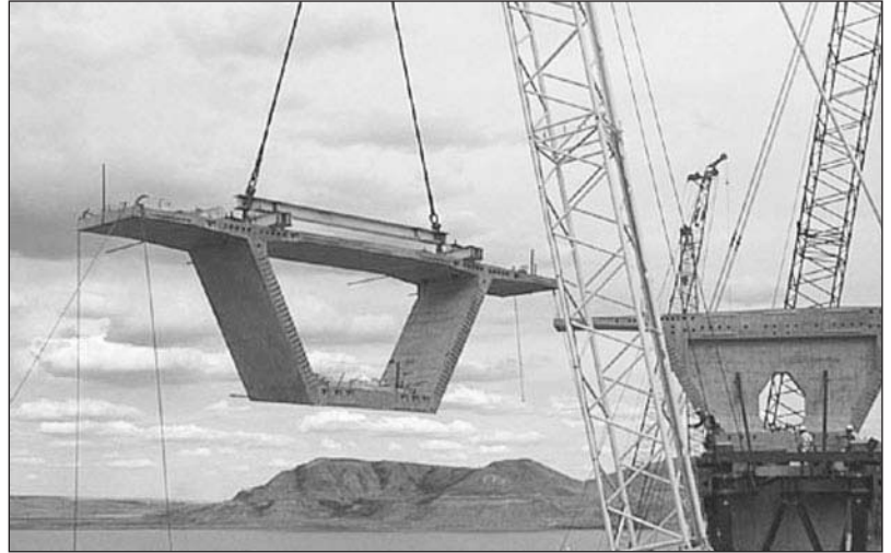
Precast concrete sections were placed to form the bridge deck.
