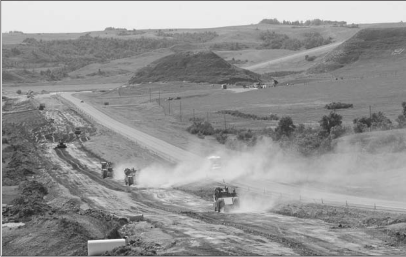
Earth work on the US 2 four-laning project near Stanley.
