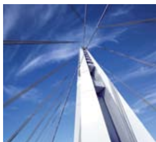
Front Cover: The main tower of the world's largest Self-Anchored Suspension Bridge will rise 525 feet above the San Francisco Bay and forever change the look of the Bay Area. This signature span is being built by American Bridge Company/Fluor Enterprises, a Joint Venture. American Bridge built the original Bay Bridge, which opened to traffic in 1936. The new bridge is scheduled for completion in 2013.
