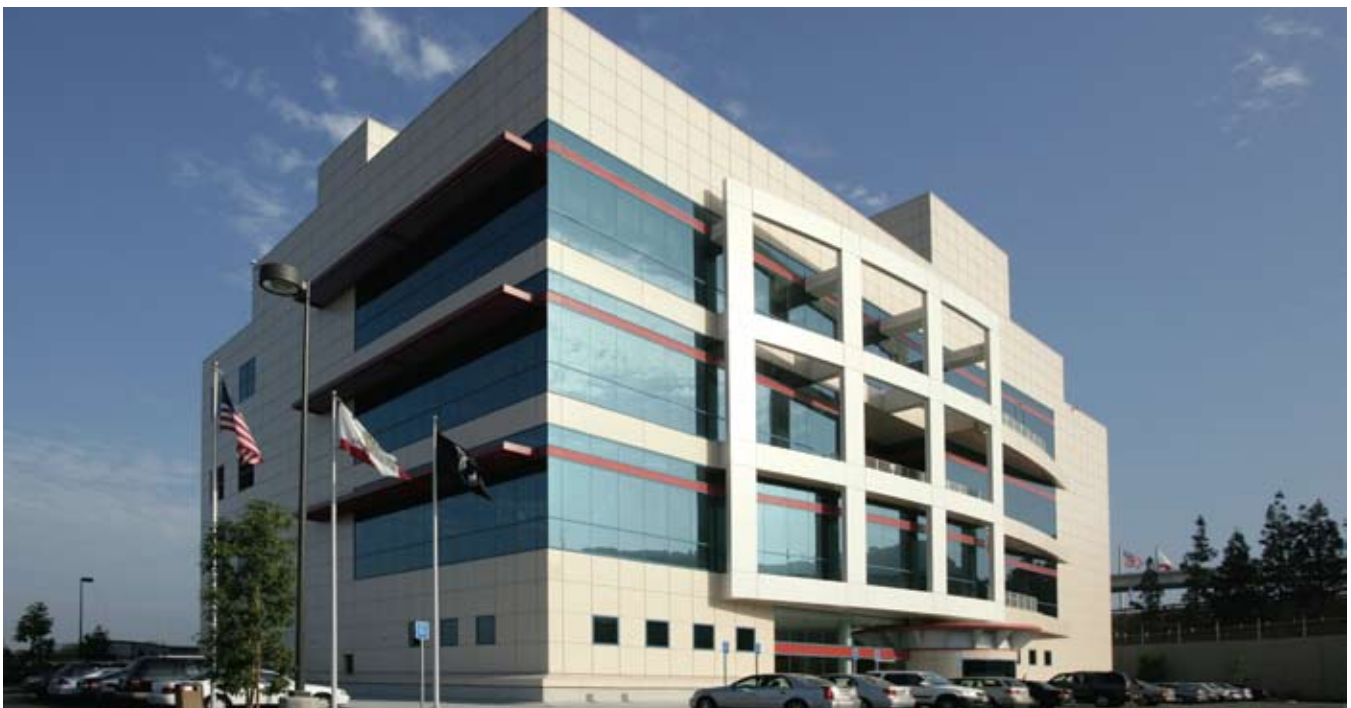
The new Los Angeles Regional Transportation Management Center opened on October 31, 2007, to serve as the hub for emergency response efforts and freeway incident management for Los Angeles and Ventura counties.
