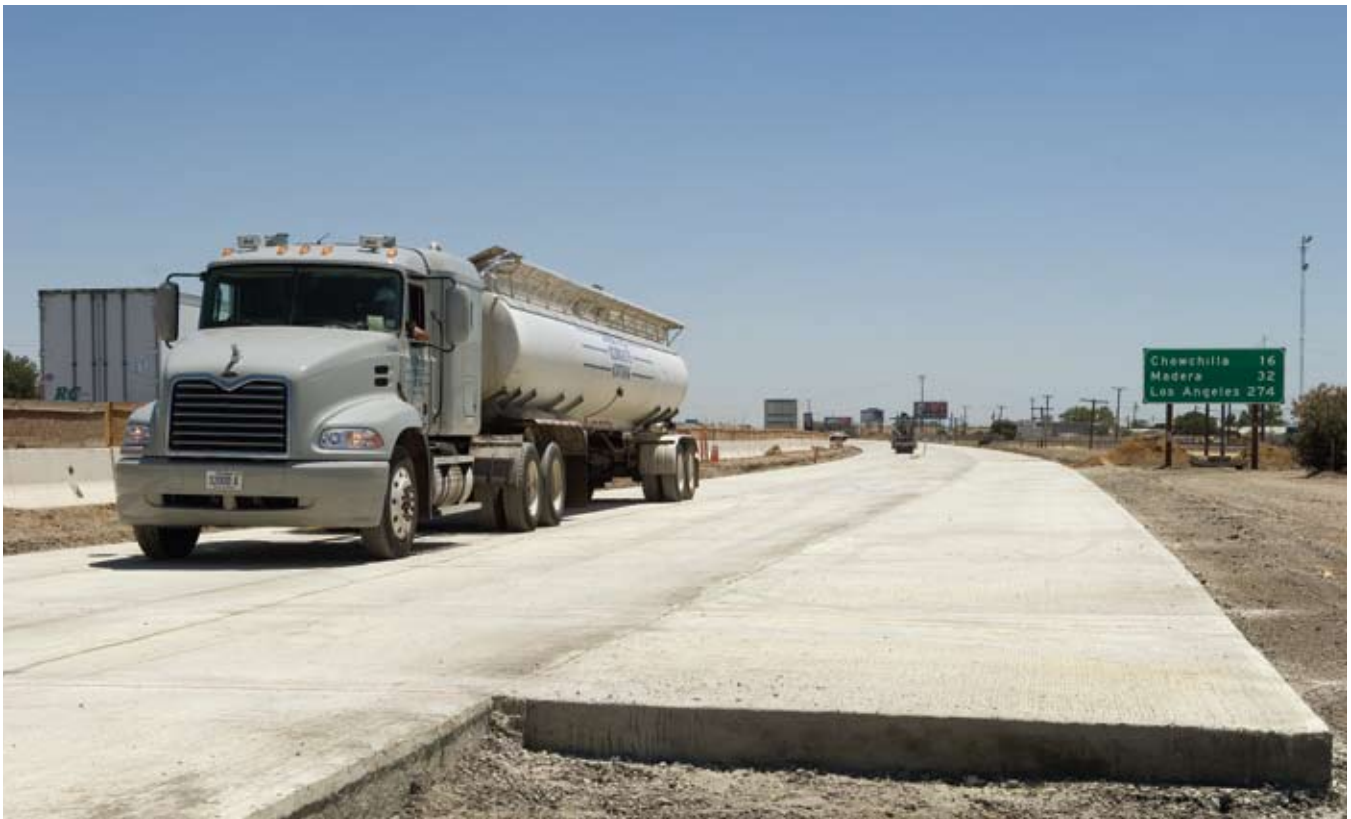
A tanker truck parks on newly constructed freeway on Highway 99 in Merced County on July 13, 2007.
