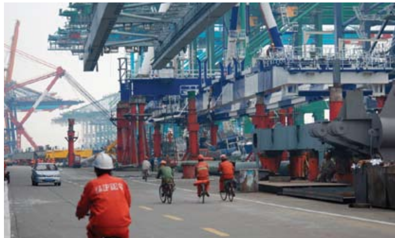
The tower and deck sections of the new Bay Bridge are being fabricated in China at the Zhenhua Port Machinery Company (ZPMC)'s facility, pictured here. ZPMC is the worldwide leader in constructing port cranes. Several cranes, as well as a shear leg barge, can be seen in the photo's background.
