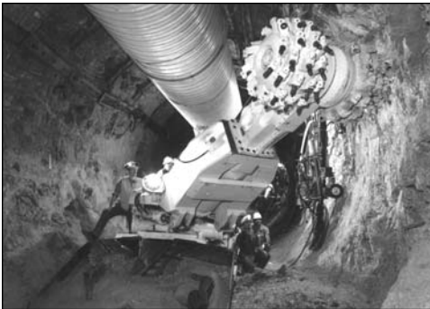
Alpine mining machines excavate alcoves for testing at Yucca Mountain
