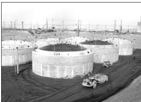
Construction of storage tanks at the Hanford Site
