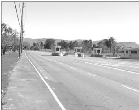
Some of the newly constructed security kiosks at Sandia
