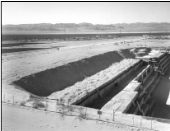
Low-Level Waste Disposal, Nevada Test Site, Mercury, NV
