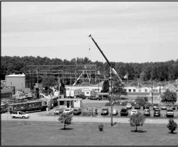
Ashtabula—Overall view of the main plant Extrusion Complex Remediation, Ashtabula, Ohio.
