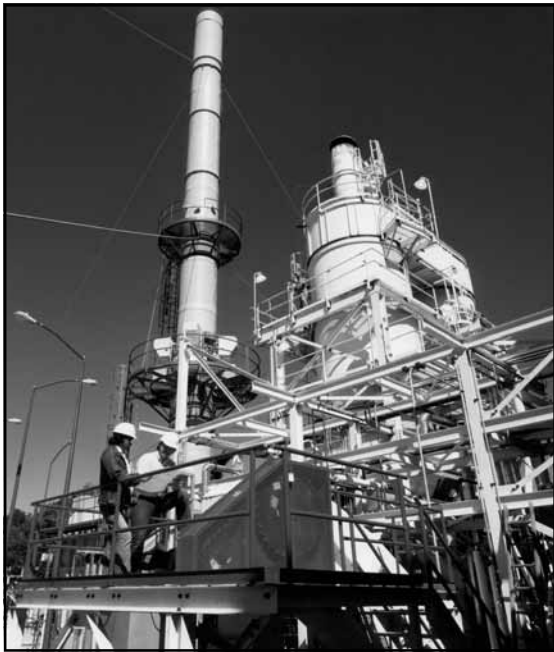
Toxic Substances Control Act Incinerator, Oak Ridge, Tennessee.
