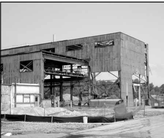
Ashtabula- Southeast corner of main plant complex, Environmental Management Project, Ashtabula, Ohio
