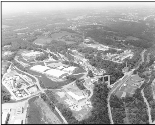
Aerial View of the National Energy Technology Laboratory (Formerly known as Pittsburgh Energy Technology Center)
