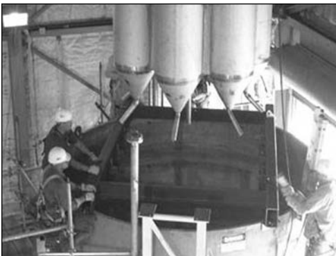
Pulse Jet Mixers used at the Waste Treatment Plant.
