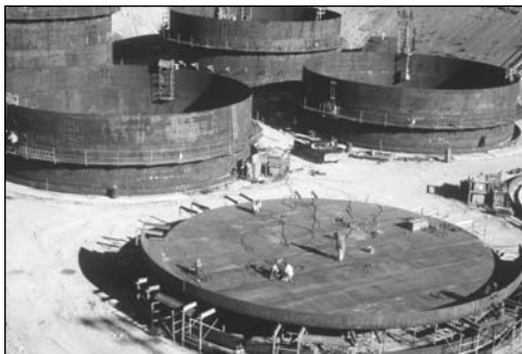
Waste storage tanks at the Hanford Site
