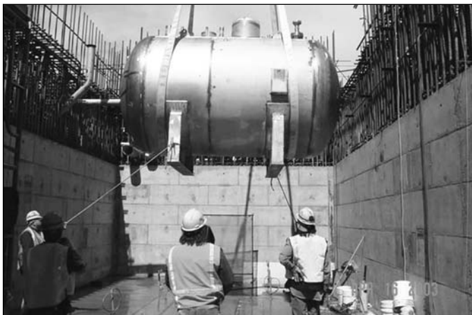
Construction of the Waste Treatment Plant at Hanford Site, Richland, WA
