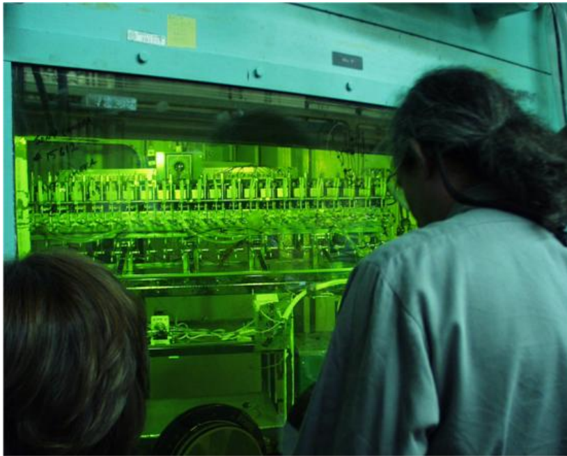
24-Stage Contactor Array used to perform the UREX+ demonstration at ANL.
