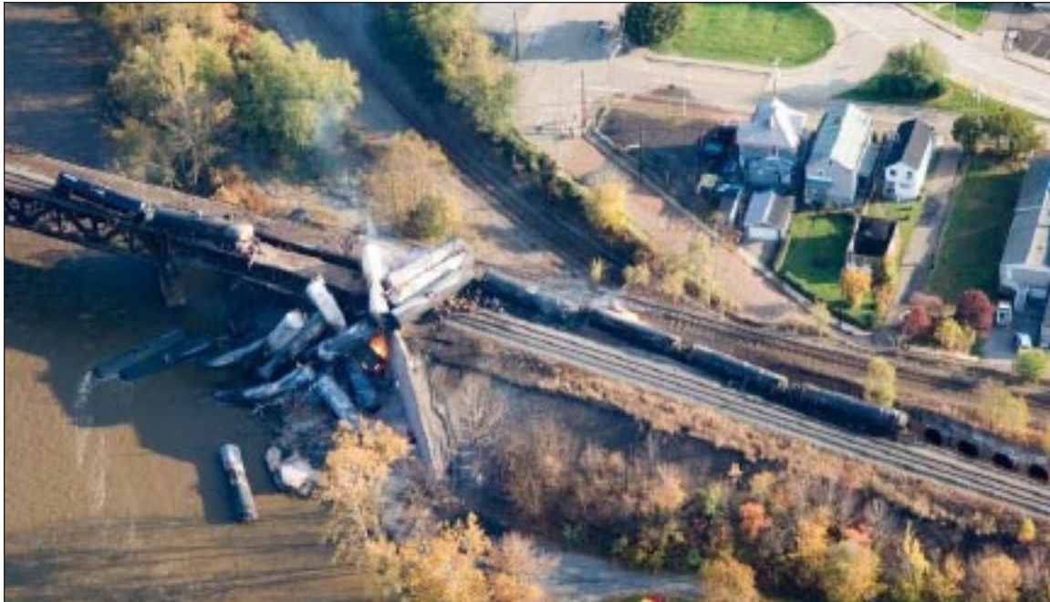
Figure 4. View of derailment showing track layout and curved track.
