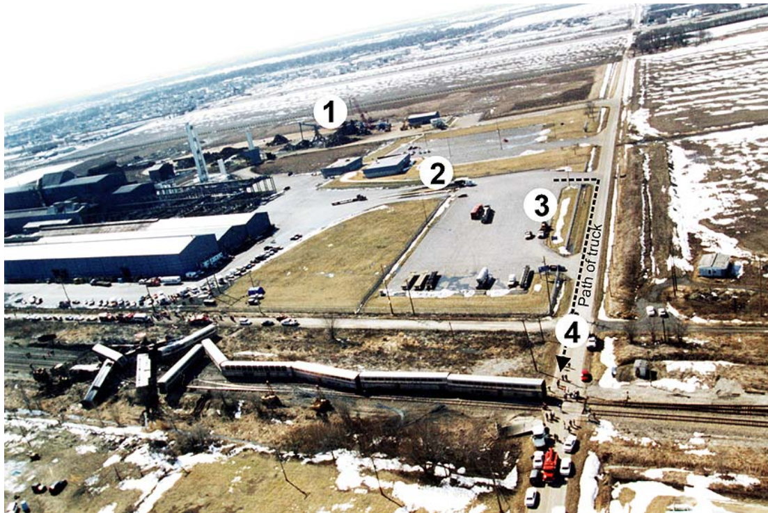
Figure 3. Aerial view of crash scene showing locations of witnesses to accident: 1. crane operator; 2. two people in scale house, 3. truckdriver affixing tarp to his load; and 4. motorist behind accident truck.
