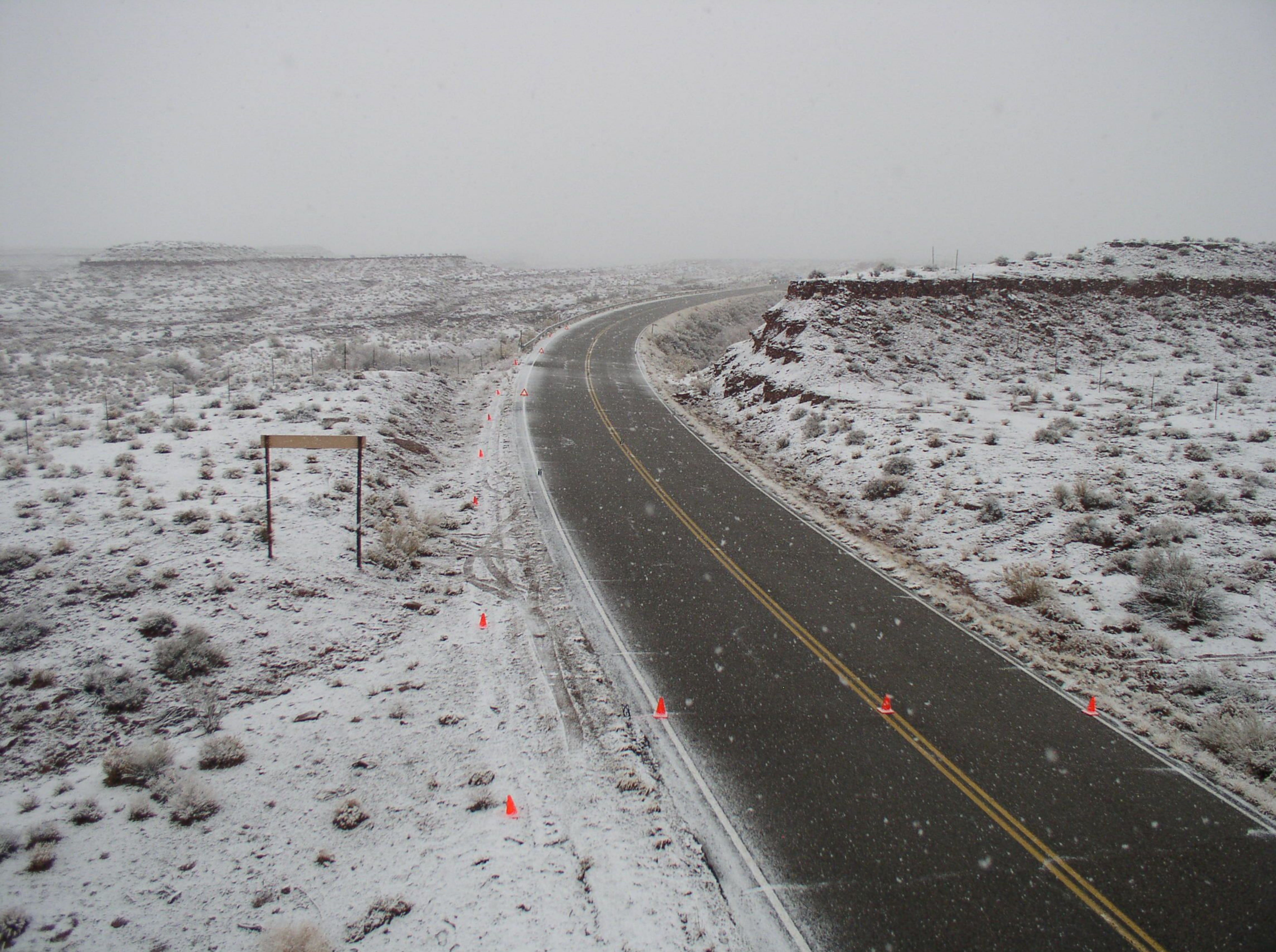
Hwy. Photo #38 - Note the distance from where the guardrail ends to the beginning of the second embankment
