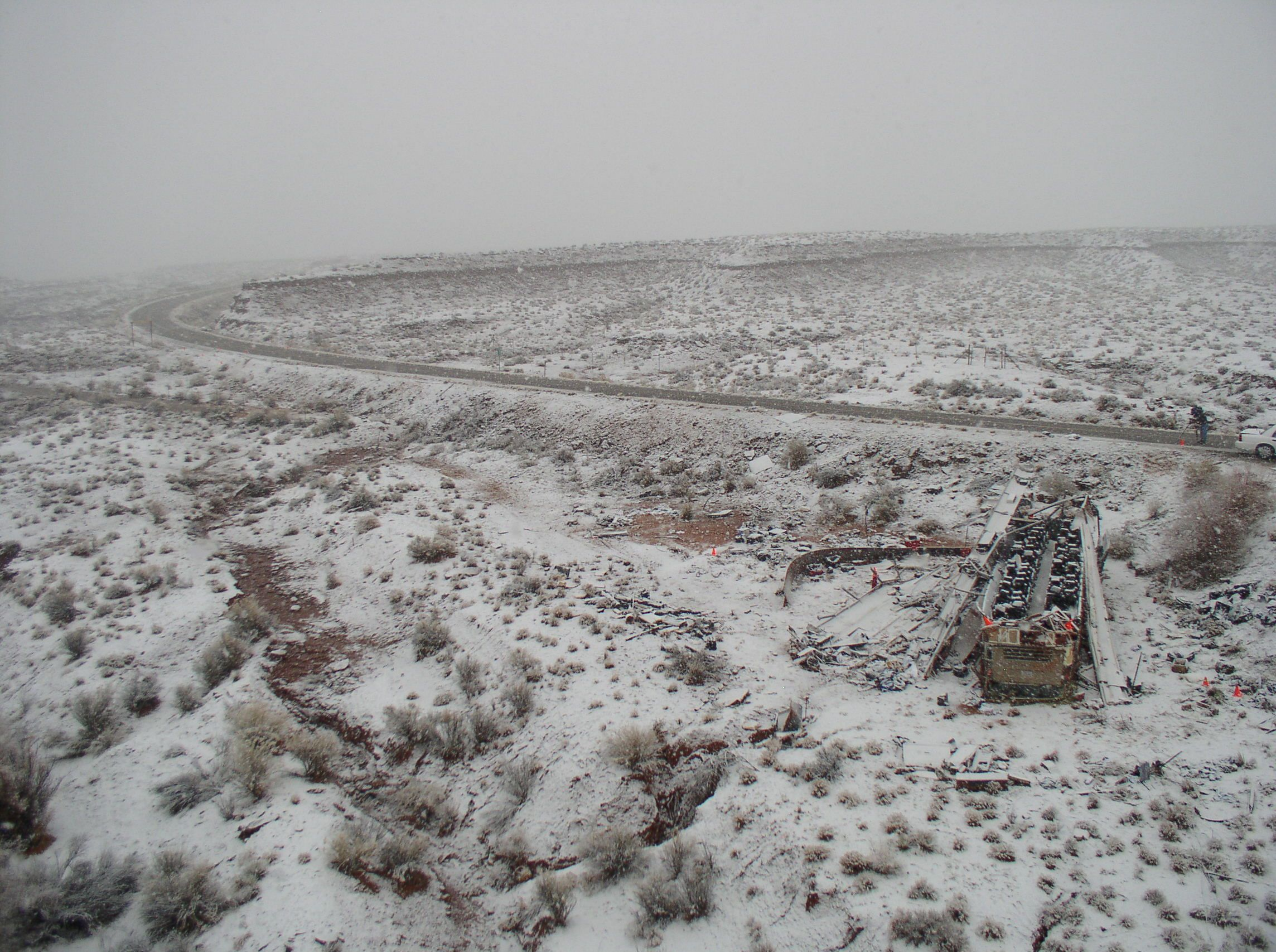
Hwy. Photo #36 - Overview of bus with embankment and curve
