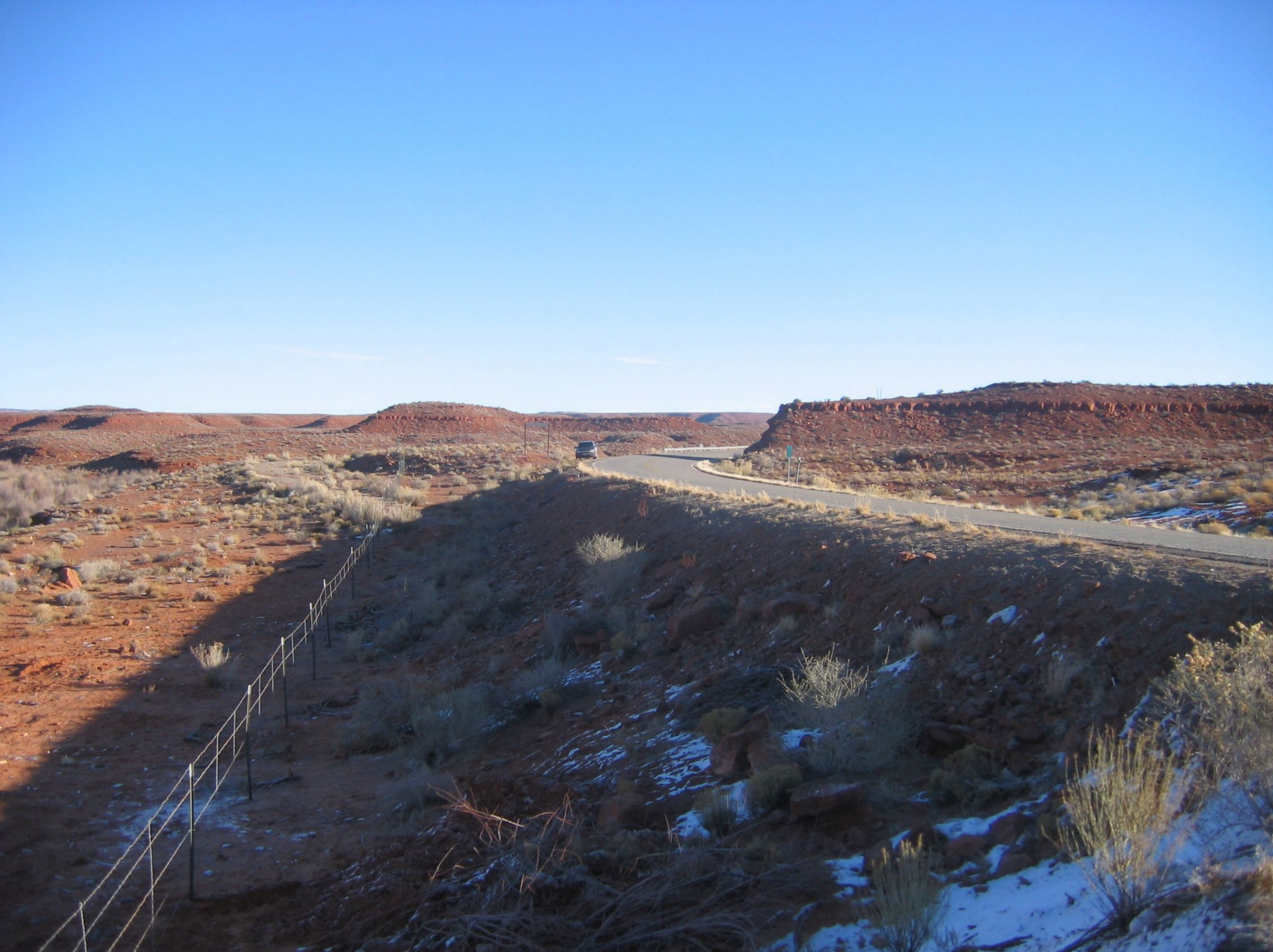
Hwy. Photo #21 - View of embankment from the opposite direction
