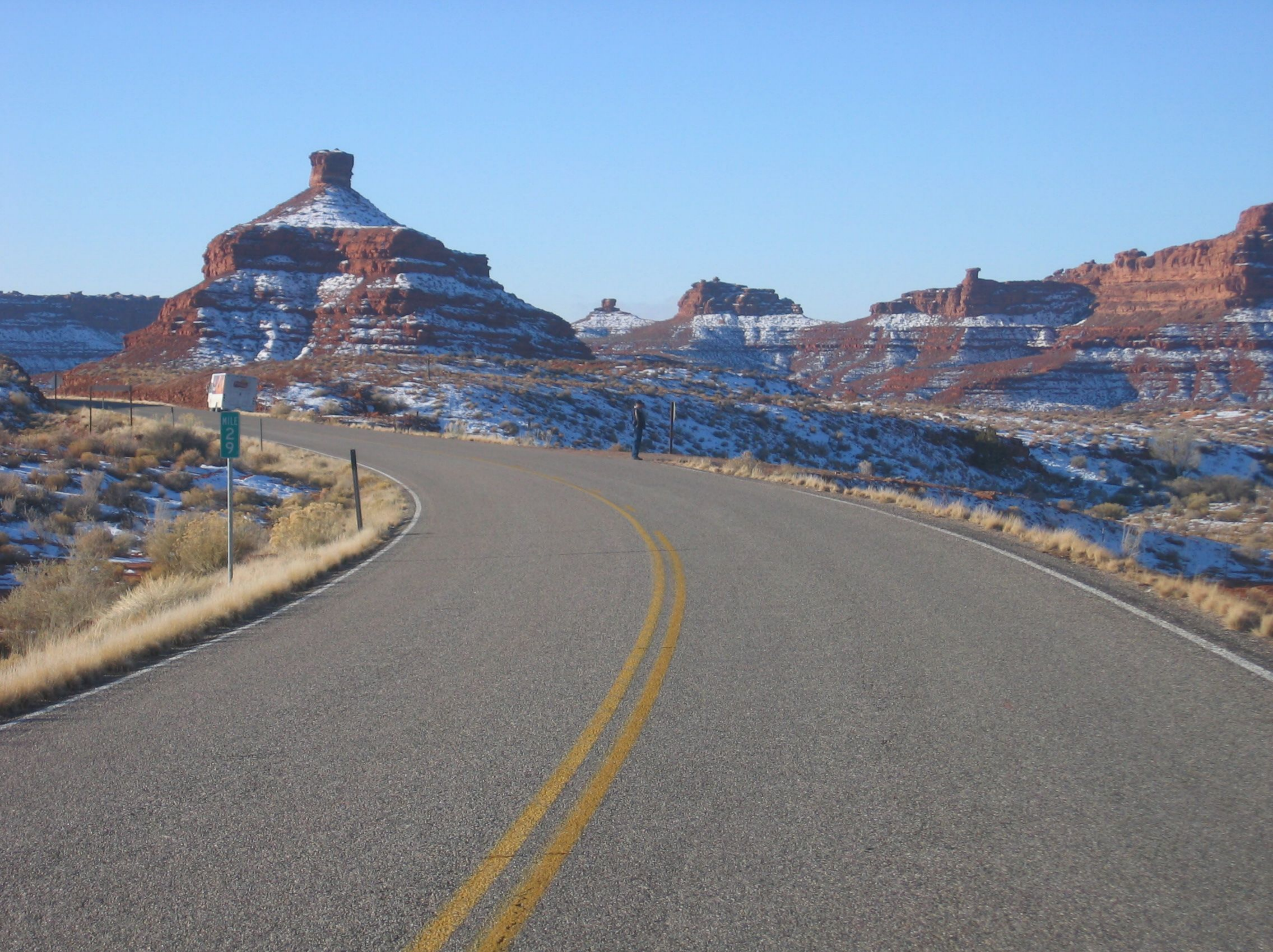
Hwy. Photo #15 - View of curve where it intersects the entrance to the "Valley of the Gods." Also, note MP marker 29 on the left-hand side
