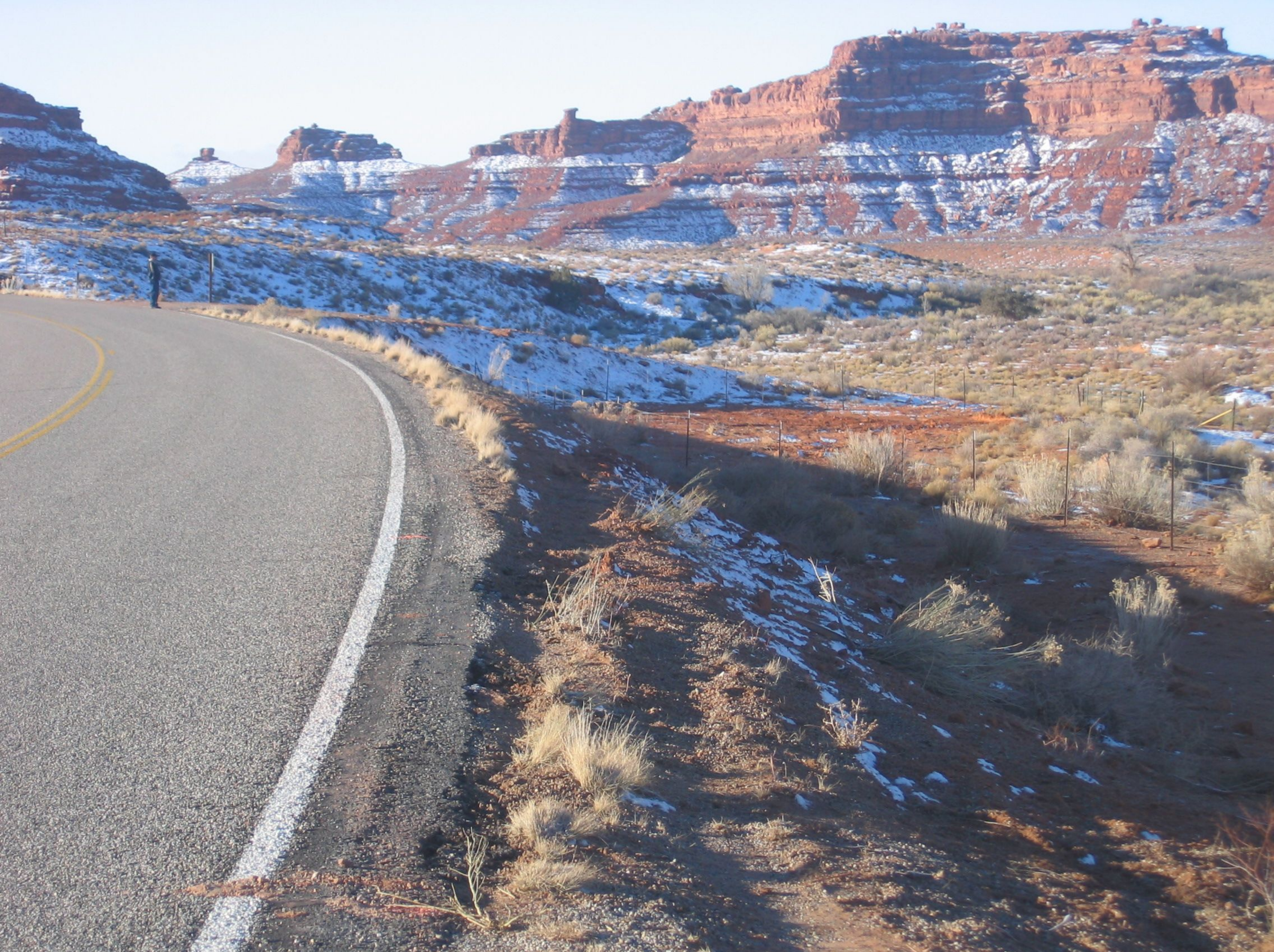
Hwy. Photo #14 - Continued view of tire marks on the beginning of the 3:1 roadside foreslope
