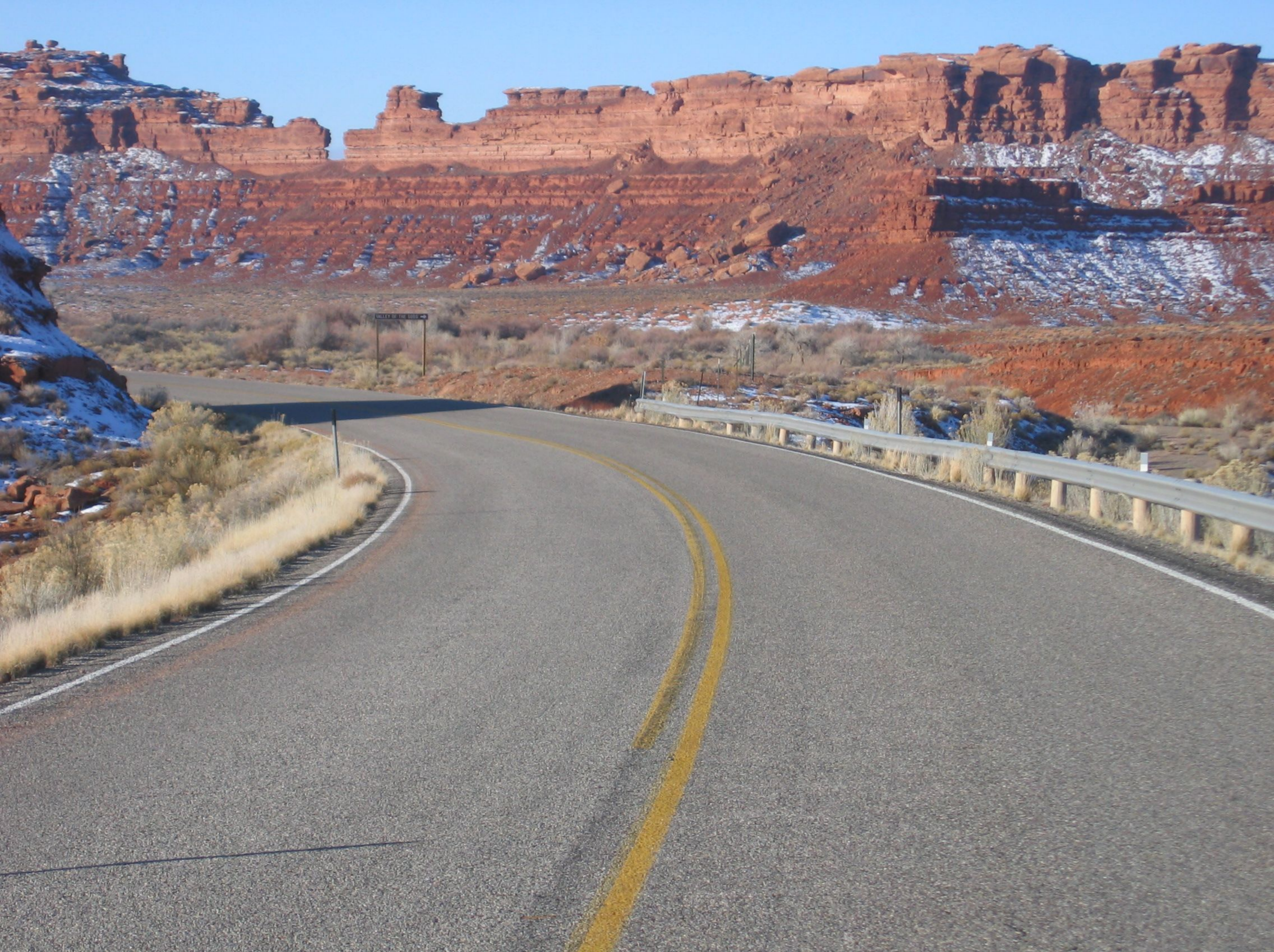
Hwy. Photo #09 - View of 4-degree 1,641-foot-long curve with guardrail ending at 772 feet into curve
