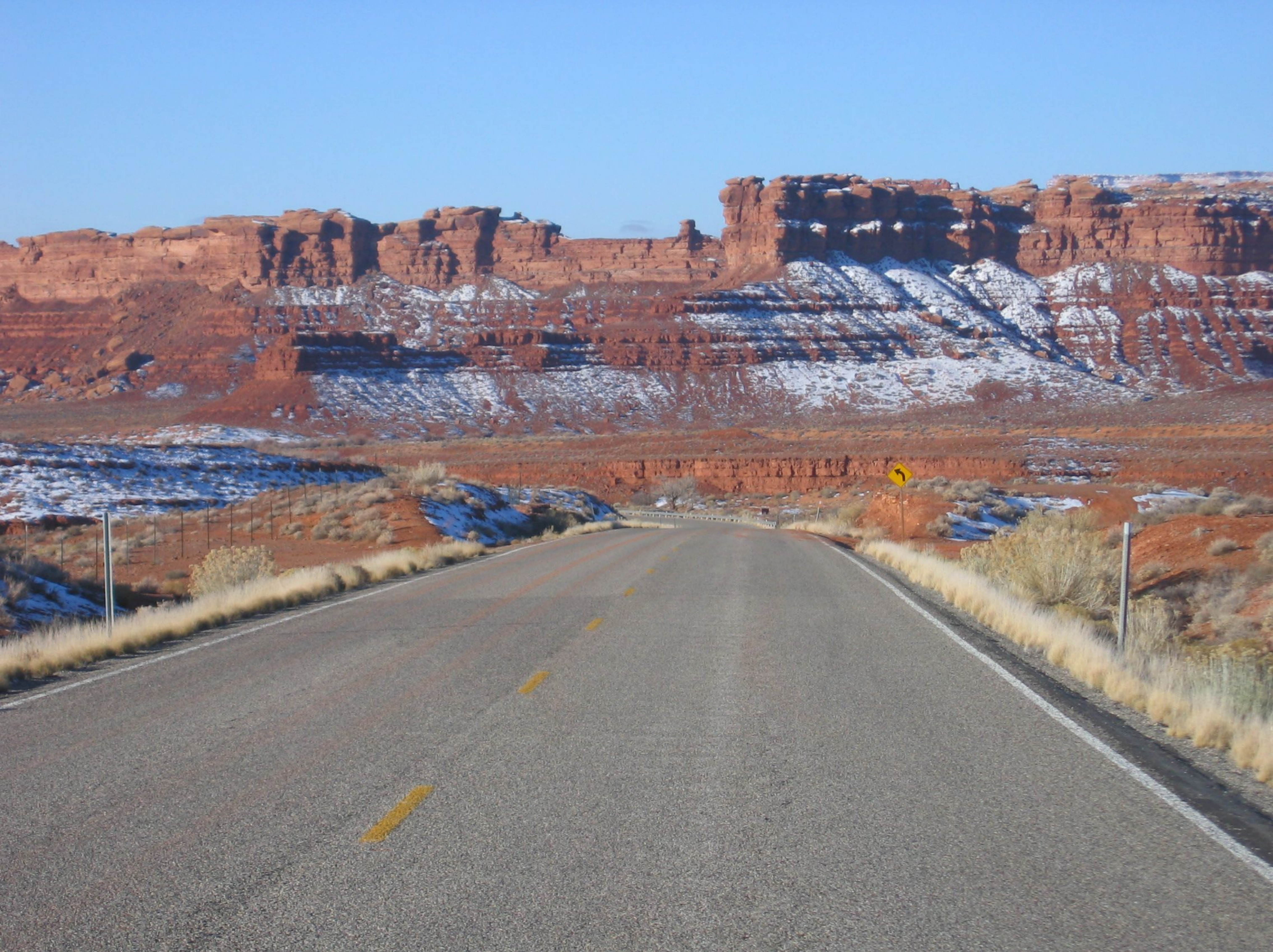
HWY. Photo #5 - View of 5.6 percent downgrade on approach to accident curve (Note the curve warning sign)
