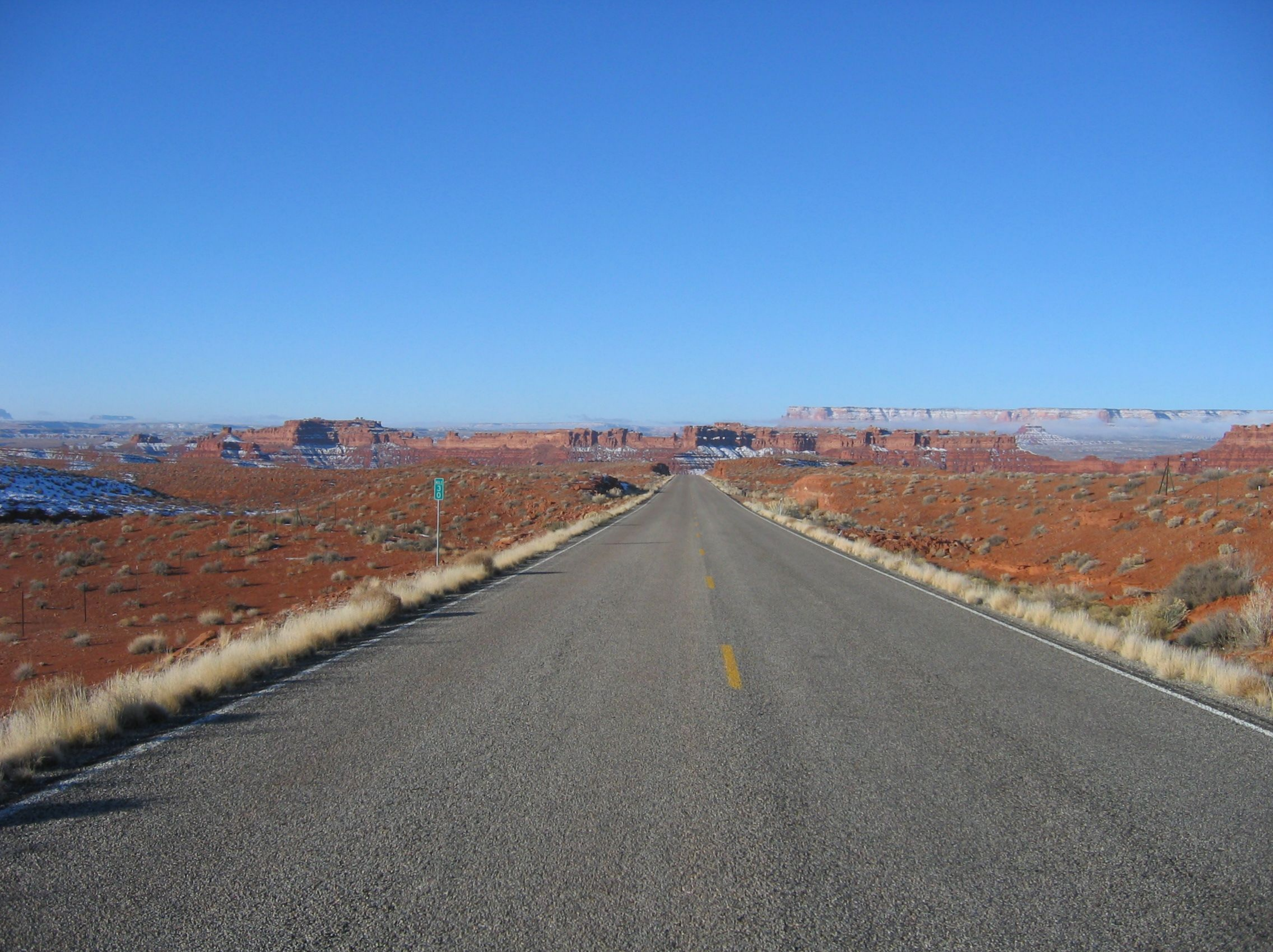
Hwy. Photo #4 - View of US 163 at MP# 30 (Average Downgrade from here to accident site is 4 percent)
