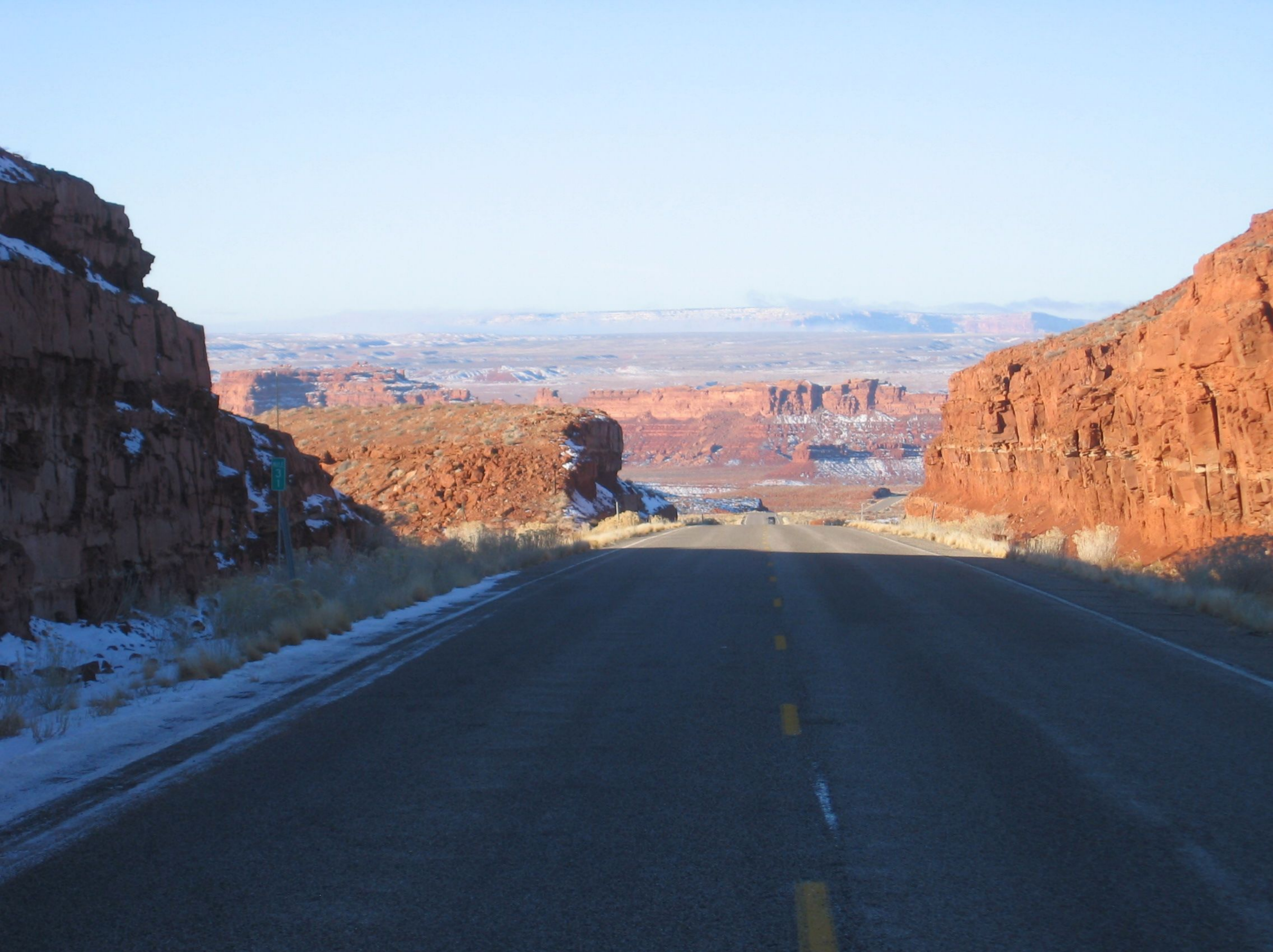
Hwy. Photo #3 - View of US 163 at MP# 31 (Notice steepness of grade)
