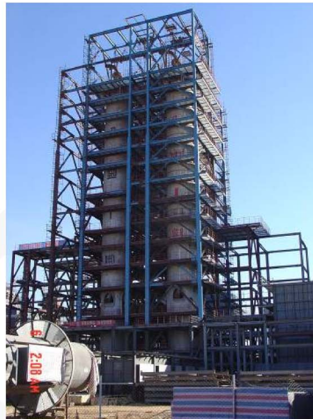
Shenhua Liquefaction Reactors
