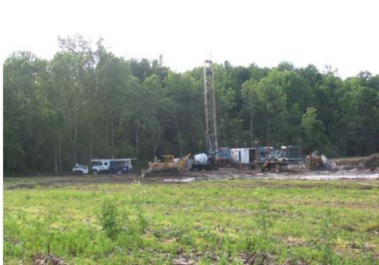
Wireline logging at Dager Well, Licking County, Ohio
