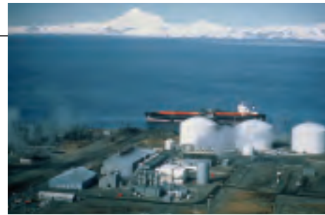
The Kenai, Alaska liquefaction facility was America's first. It has exported LNG to Japan for more than 30 years.
