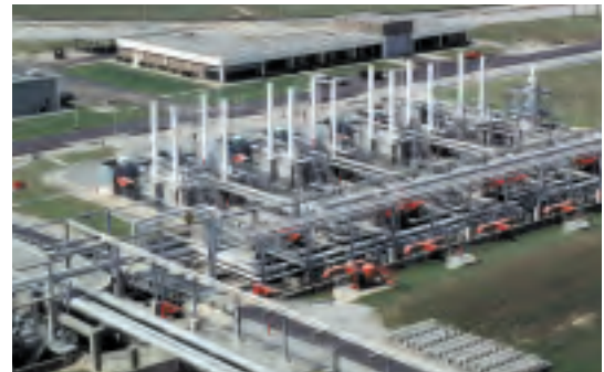
Regasification system at the Lake Charles, Louisiana LNG terminal
