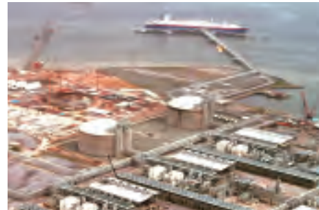
After liquefaction, the LNG is stored in insulated tanks until it can be loaded onto carrier ships. This photo shows such tanks in Trinidad and Tobago.
