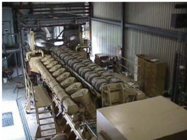
Figure 5: Picture of the Fairbanks Morse Coal Diesel Engine Installed at UAF
