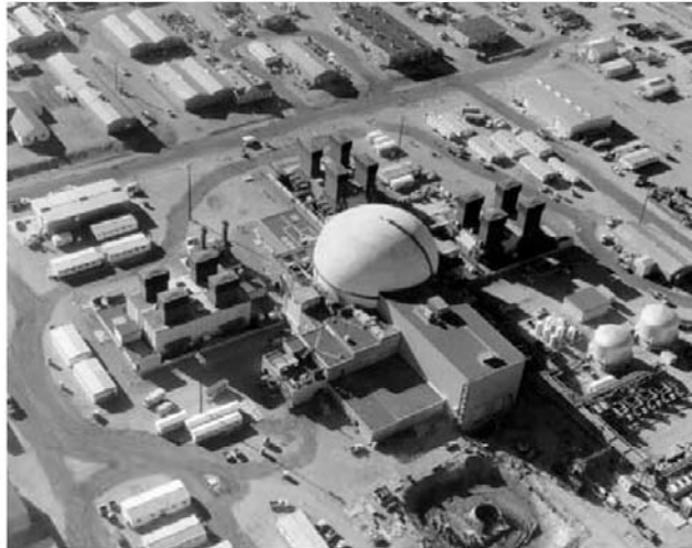
FFTF was the last large operating U.S. fast reactor.
