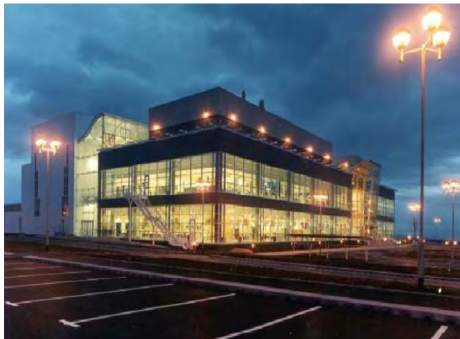
Figure 2-1. The British Technology Centre is a new facility with advanced fuel cycle development capabilities.
