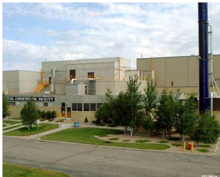
Fuel Conditioning Facility at the Idaho National Laboratory
