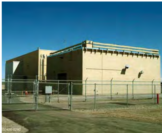
Space and Security Power Systems Facility at the Idaho National Laboratory
