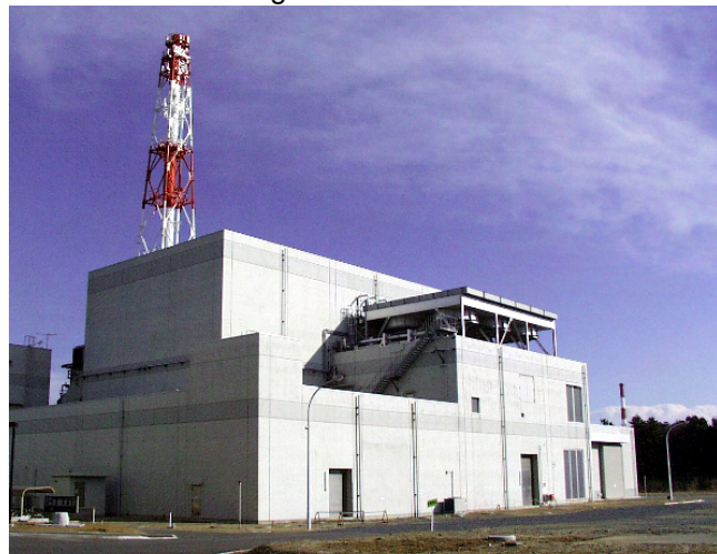
The High Temperature Engineering Test Reactor in Japan
