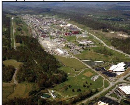
Y-12 National Security Complex
