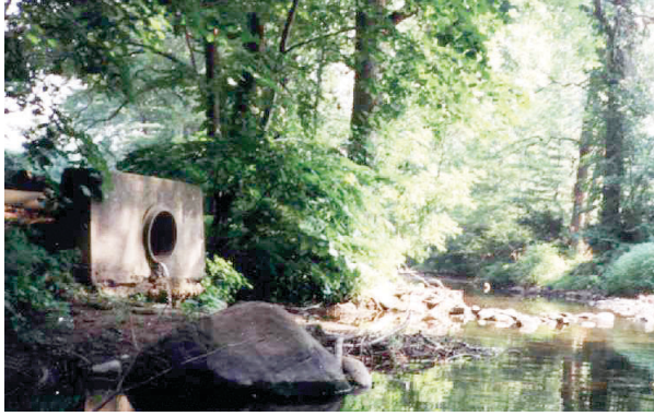
Figure 14. Unregulated impervious-area runoff exemplified by a storm-sewer pipe that drains directly into the Saddle River at Ridgewood, N.J. (01390500).
