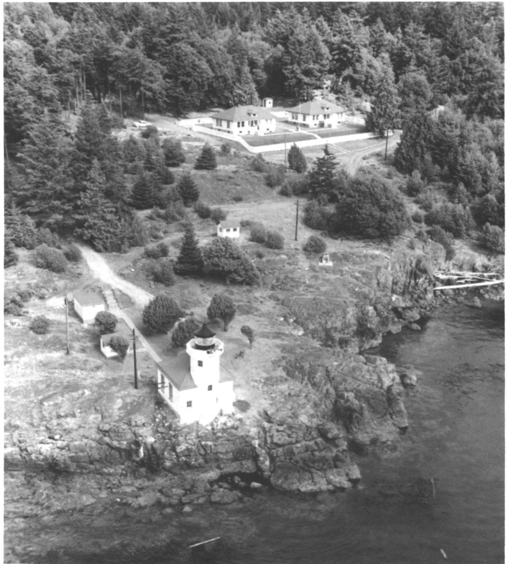
The Lime Kiln Light Station marks an eastern point on Hard Strait in the Puget Sound of Washington. The complex, consisting of the light and fog signal building, the keeper's and assistant keeper's dwellings, the shop, and the oil and coal house, is unique because the entire station was designed concurrently in 1917. Furthermore, all the buildings are made of reinforced concrete, an early use of this material for buildings of such varied functions. Lime Kiln is the first and only known example in the Pacific Northwest of such extensive use of the material; virtually every major lighthouse built in this area since 1917, has been made of concrete. (U.S. Coast Guard)
