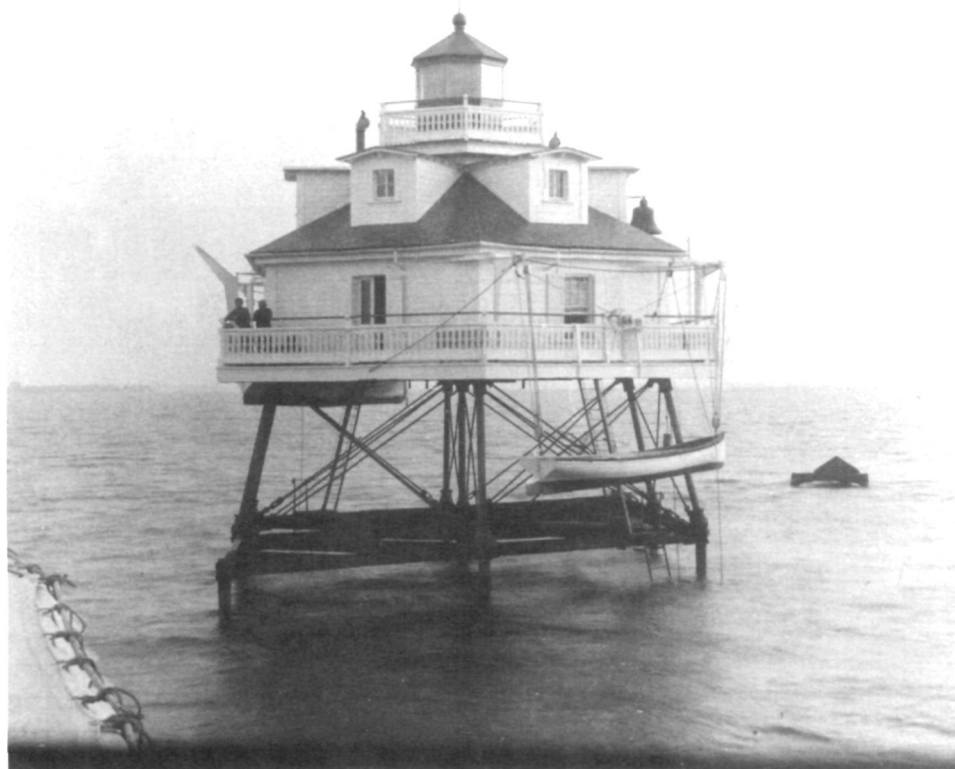
Thomas Point Shoals Light Station, standing in Maryland's Chesapeake Bay, is a hexagonal screwpile, offshore light. Screwpile refers to the nine metal pilings, tipped with two blades arranged in screw fashion, which support the structure. This method of anchoring an aid to navigation was most appropriate for the sandy, muddy bottom of the bay. In this historic photograph, taken in 1885, ten years after the completion of the light, its roof is topped with dormers and a steel octagonal cupola containing the light. (U.S. Coast Guard)
