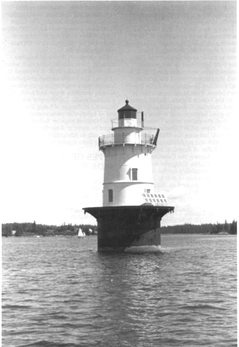
The Goose Rocks Light Station marks the east entrance to the Fox Island thoroughfare between Vinalhaven and North Haven Islands in Maine. The caisson or sparkplug light, constructed in 1890, stands on a shallow rock ledge. Within its walls are the keeper's quarters and the storage facility. The light guides not only cargo ships but pleasure vessels as well. The two islands attracted many summer tourists with numerous hotels and cottages built to serve the growing resort communities. (Roger G. Reed)
