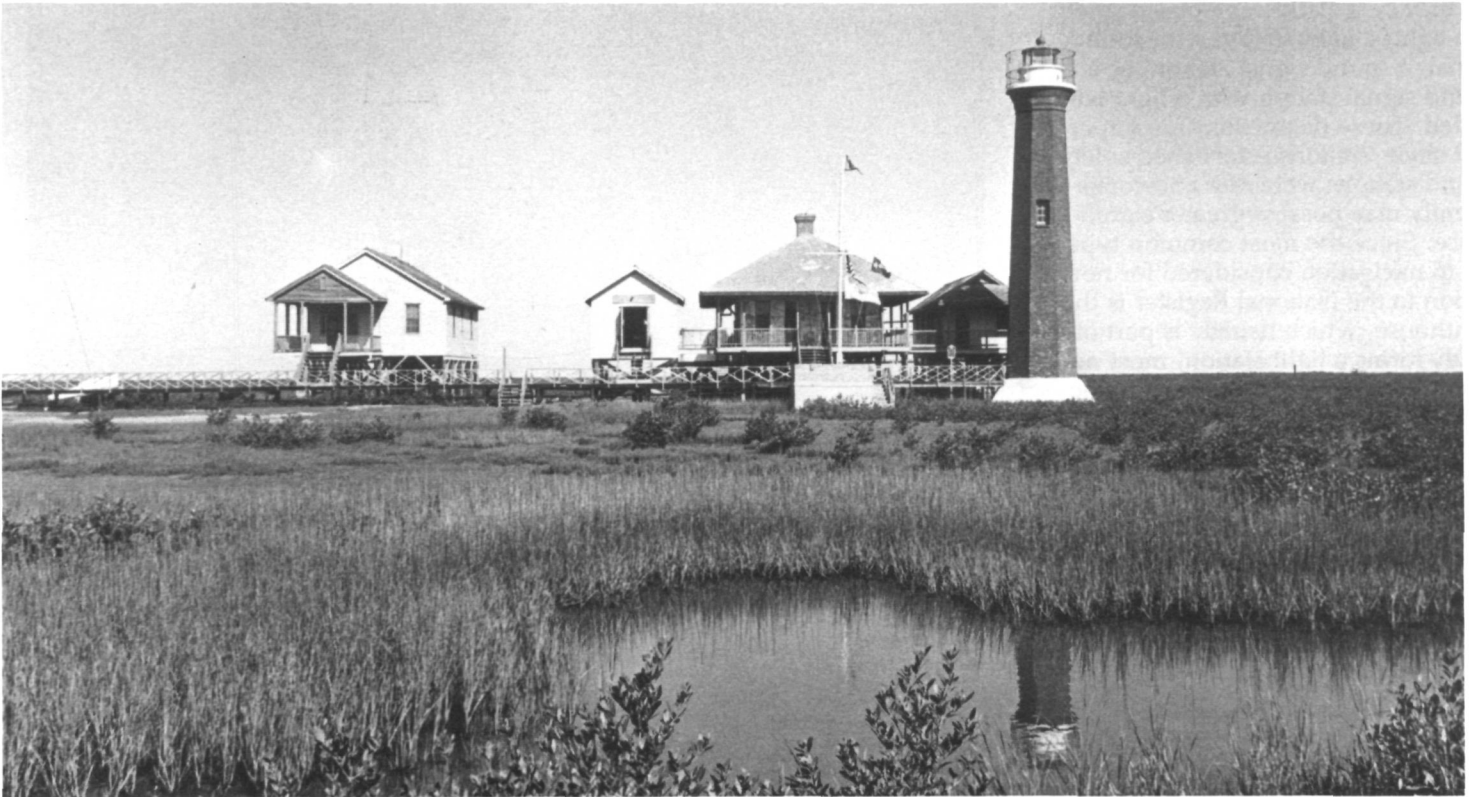
The Aransas Pass Light Station is the second oldest lighthouse on the Texas coast. First lighted in 1857, the station exhibited its beam from the top of a cylindrical brick tower that remained unpainted. A white light emanated from a fourth order, fixed Fresnel lens. During the Civil War, the tower was a daymark for blockading Federal vessels as well as a viewing platform for Union sailors. In December 1862, Confederate soldiers blew off its top with black powder. Relighted in 1867, the light guided shipping along the Texas coast. (Kay Franklin)
