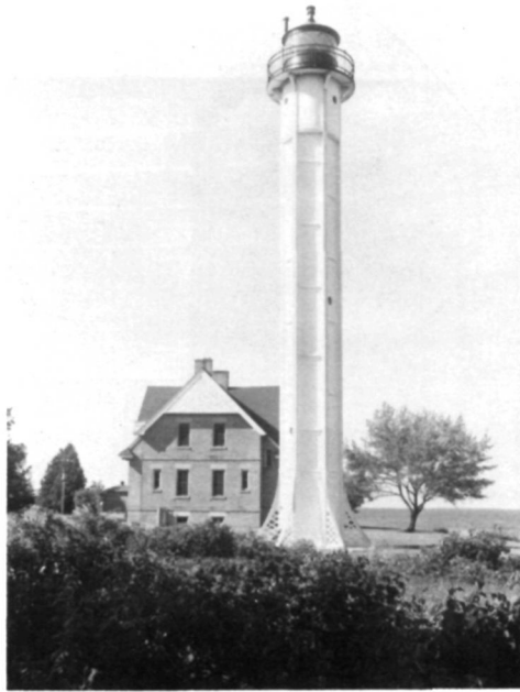
The light tower of St. Martin Island in Michigan is an excellent example of a pure exoskeletal tower on the Great Lakes. The six-sided tower is supported by six exterior steel posts which have latticed buttresses. The Fourth Order Fresnel lens consists of two glass panels separated by a brass reflector so that when turned, the lens produces alternating red and white flashes. (U.S. Coast Guard)
