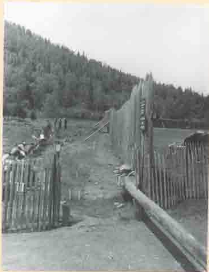
Excavations along exterior of Western palisade
