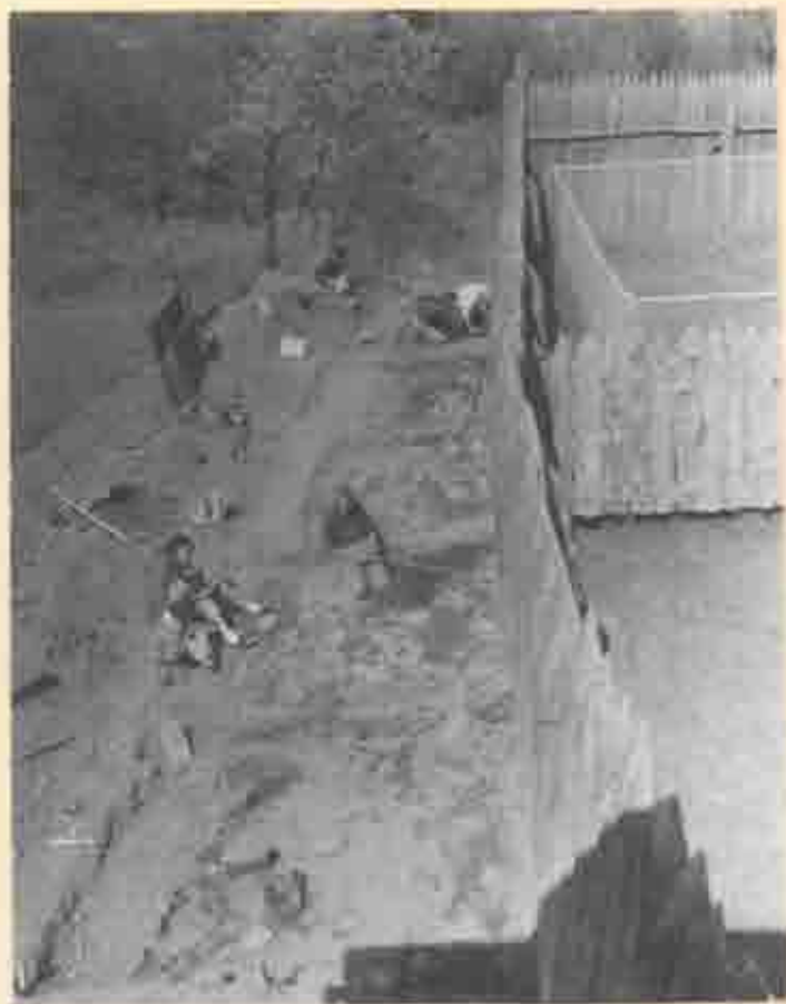
Excavations, Corners G to H, 1966
