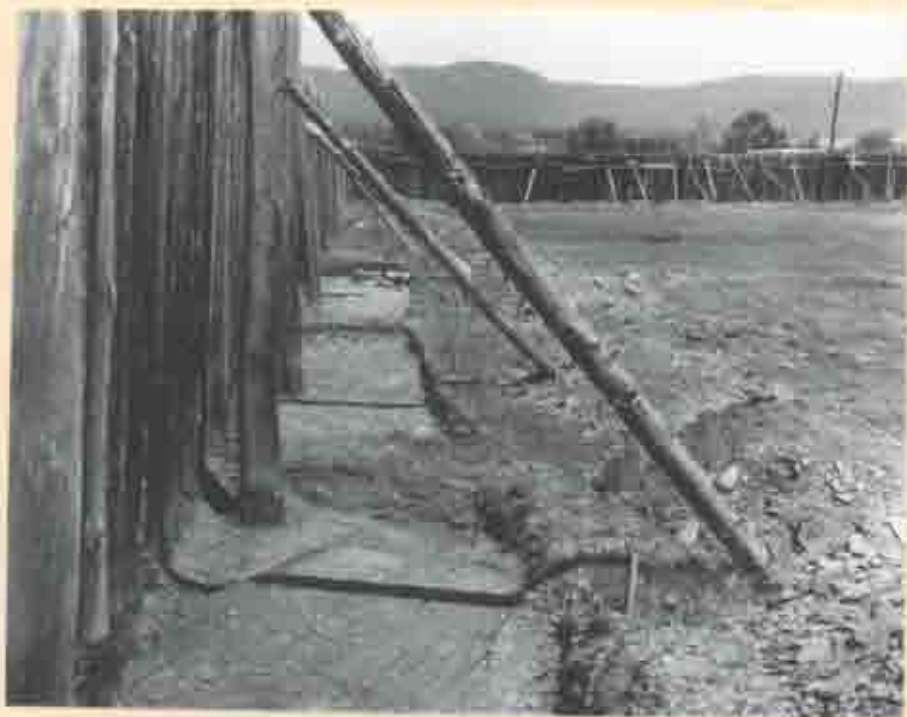
Excavation along interior of Northern palisade
