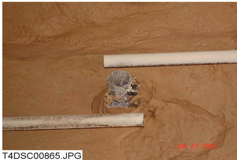
Figure 3-121. Drain collar surrounded by sediment on the tank bottom.
