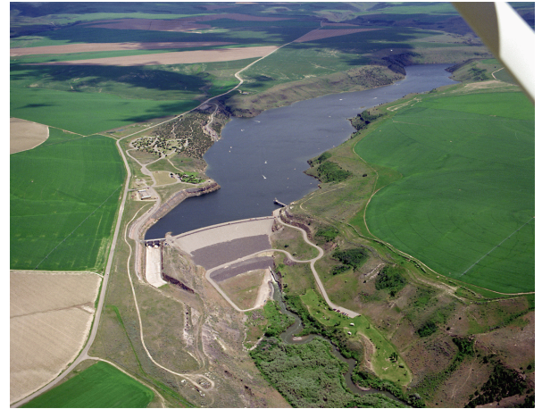
Photo 3-2. Juniper Park is located upstream of Ririe Dam; Creekside Park is located immediately downstream.
