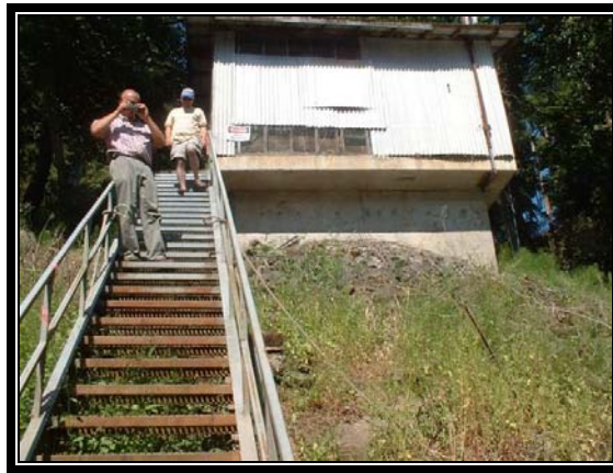
Photograph 3. West view from intake showing pump house.
