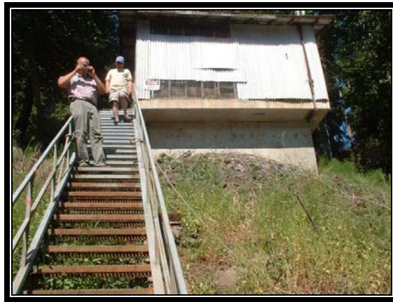
Photograph 3. West view from intake showing pump house.
