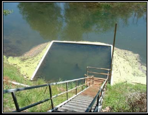
Photograph 2. East view of existing intake at base of slope.
