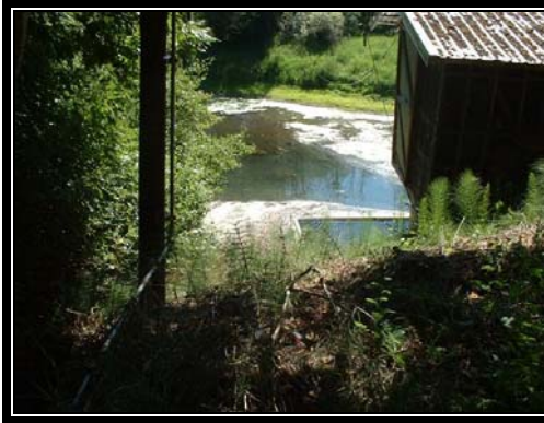
Photograph 1. East view of existing pump house. Intake at base of slope.
