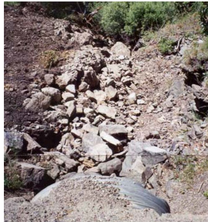
Figure 2-10. Example of backfill and riprap armament with minimal concrete and metal components
