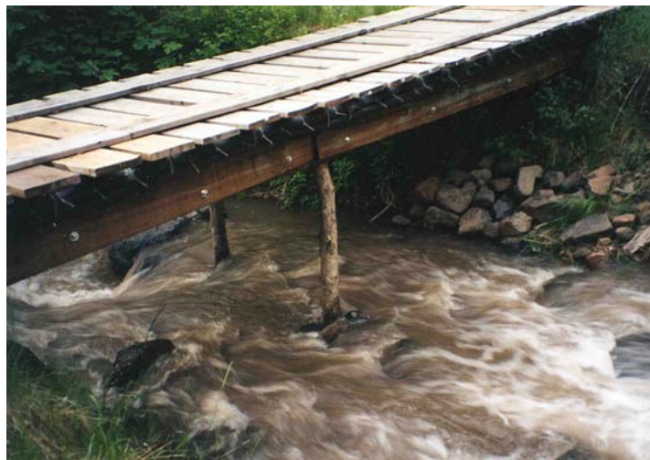
Figure 2-12. Bridge site where standard engineering techniques would be beneficial
