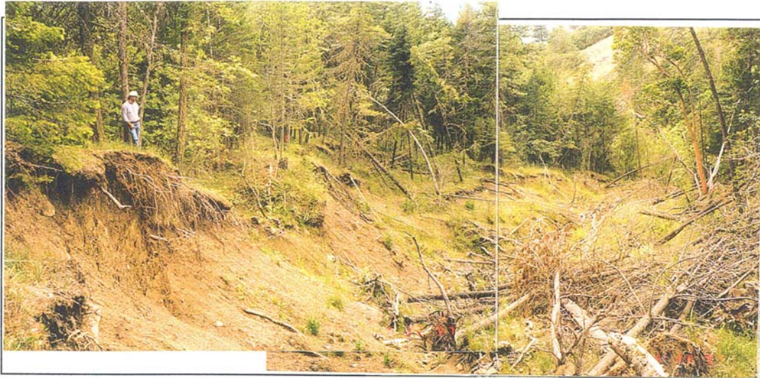
Panoramic Photograph No. 7. Tyler Creek Wasteway. Looking downstream from about Station 60+70 to 64+40. Photograph shows acute erosion in altered/weathered fine-grained volcanics with very few hard rock clasts exposed. Toppled trees are a result of bank undercutting. Note landslide topography in center of photograph. Maximum height of eroded bluffs is about 40 feet. USBR Photograph by B.H. Carter, 6/26/97.
