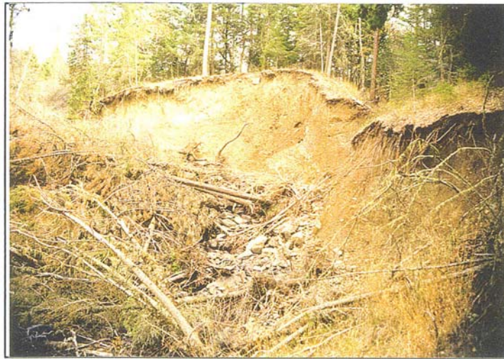
Photograph No. 9. Tyler Creek Wasteway. This photograph was taken in November 16, 1993 when the recent channel erosion had formed near vertical bluff to 40 feet in height. In comparison with Photograph No. 8 taken in 1997, note the bluff exposures have migrated upslope producing flatter slopes.
