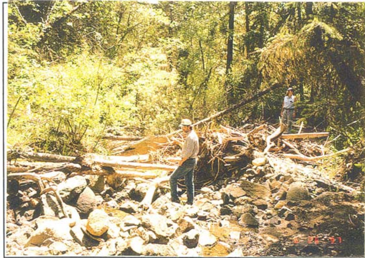
Photograph No. 5. Tyler Creek Wasteway. Looking downstream (southwest) at channel mantled with hard, volcanic gravel to boulder-size materials; Station 54+34. Channel area is well armored with tree/rock bar causing flow obstruction and lateral migration of streamflow. USBR Photograph by B.H. Carter, 6/26/97.
