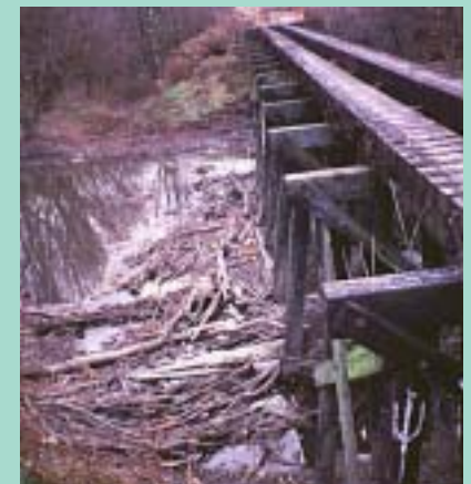
Allowing trash, logs or debris to collect at choke points can dam up a channel.
