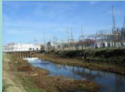
This private utility's critical facility is in a floodway.
