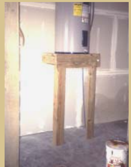
Wet floodproofed garage in Wrightsville Beach, NC.
