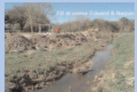
Encroachments in the floodway cause increases in flood elevation, both upstream and downstream.
