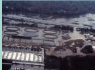
Wastewater treatment plants are often located in floodplains, or worse yet, floodways and subject to damage, causing pollution.
