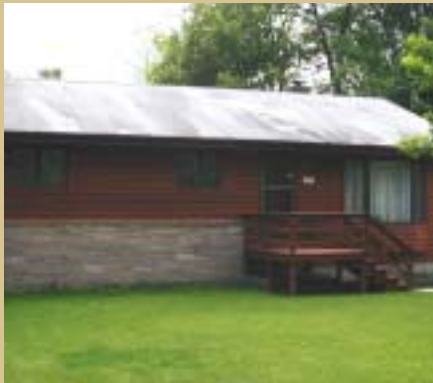
This Illinois home was elevated one foot above the base flood elevation in a shallow floodplain. The site has been flooded several times since the project was completed, but water did not damage the home.
