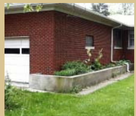
Barriers close to the building will have a minimal impact on loss of flood storage, but still must account for openings (Calumet City, IL).
