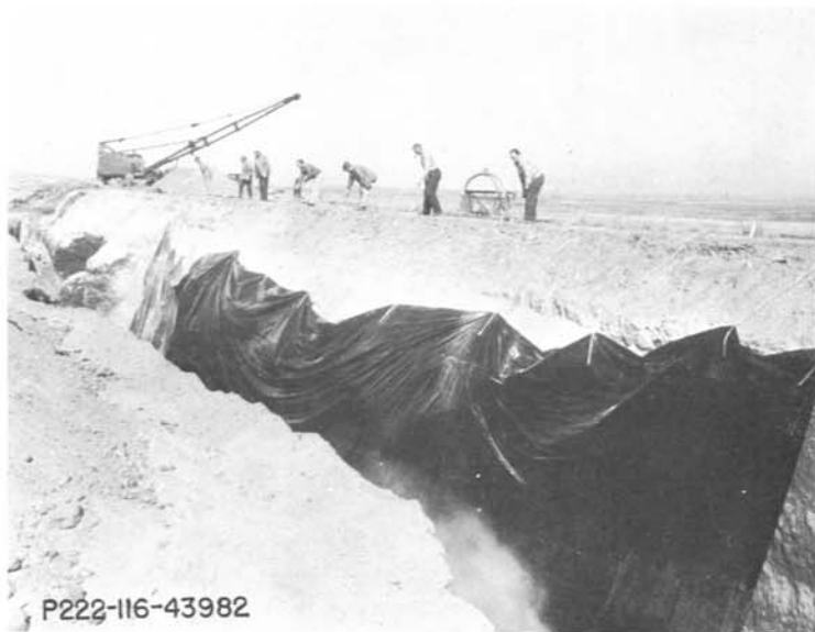
Figure 4 shows workmen placing the plastic sheet in the reach shown previously. Although the filament tape anchored to the upper edge of the plastic was spaced 10 to 12 feet apart, it appeared to be quite secure. Additional anchors were placed to strengthen the hold on the plastic after it was determined the plastic was being subjected to considerable stress during subsequent backfilling operations.
