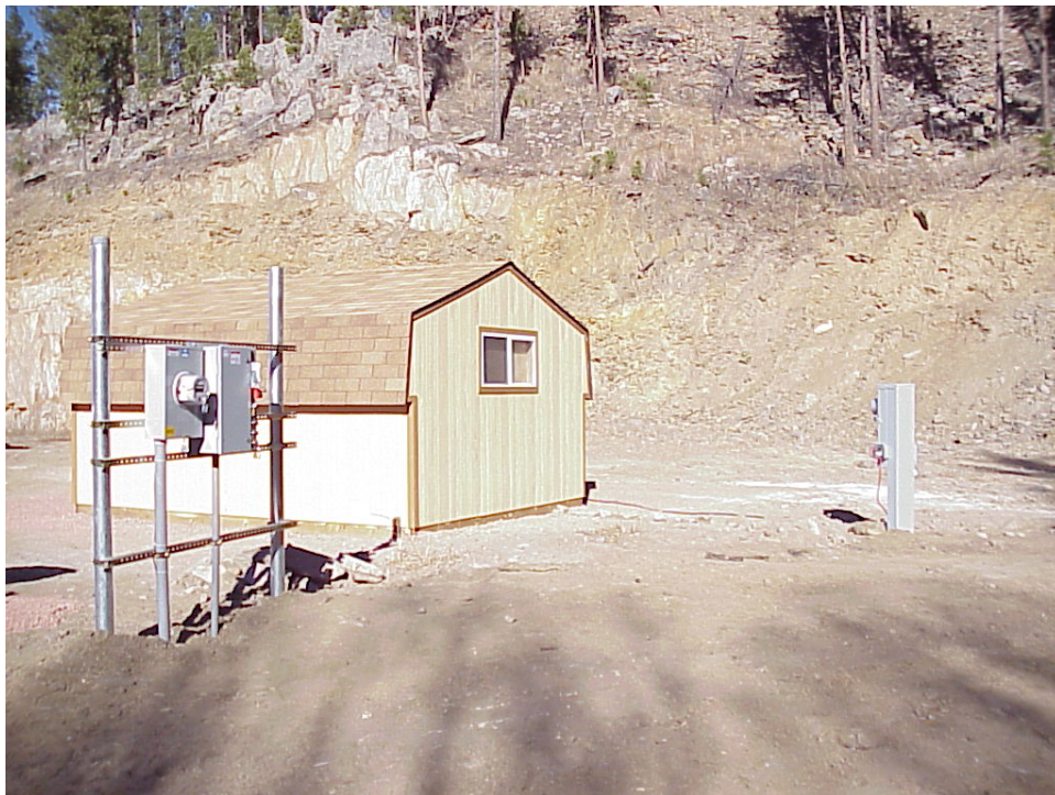
Figure 5. Keystone City Well No. 4.
