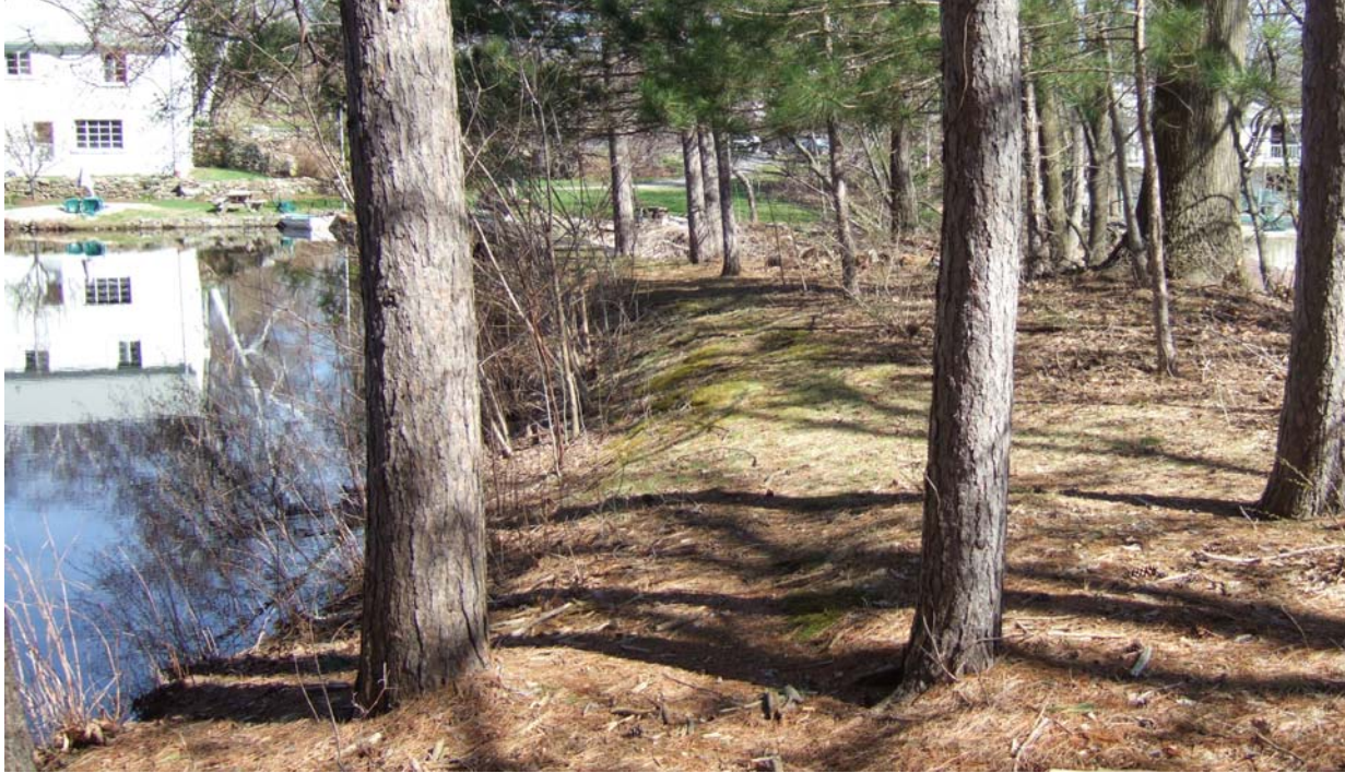
Figure 4. 4 Earth Embankment of the Hughesdale Lower Pond Dam
