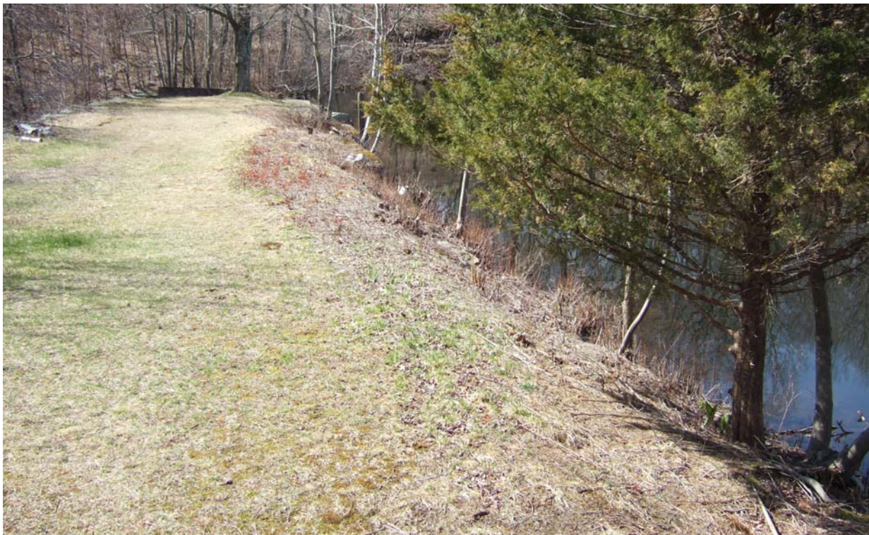
Figure 4. 7 Earth Embankment of the Hughesdale Upper Pond Dam
