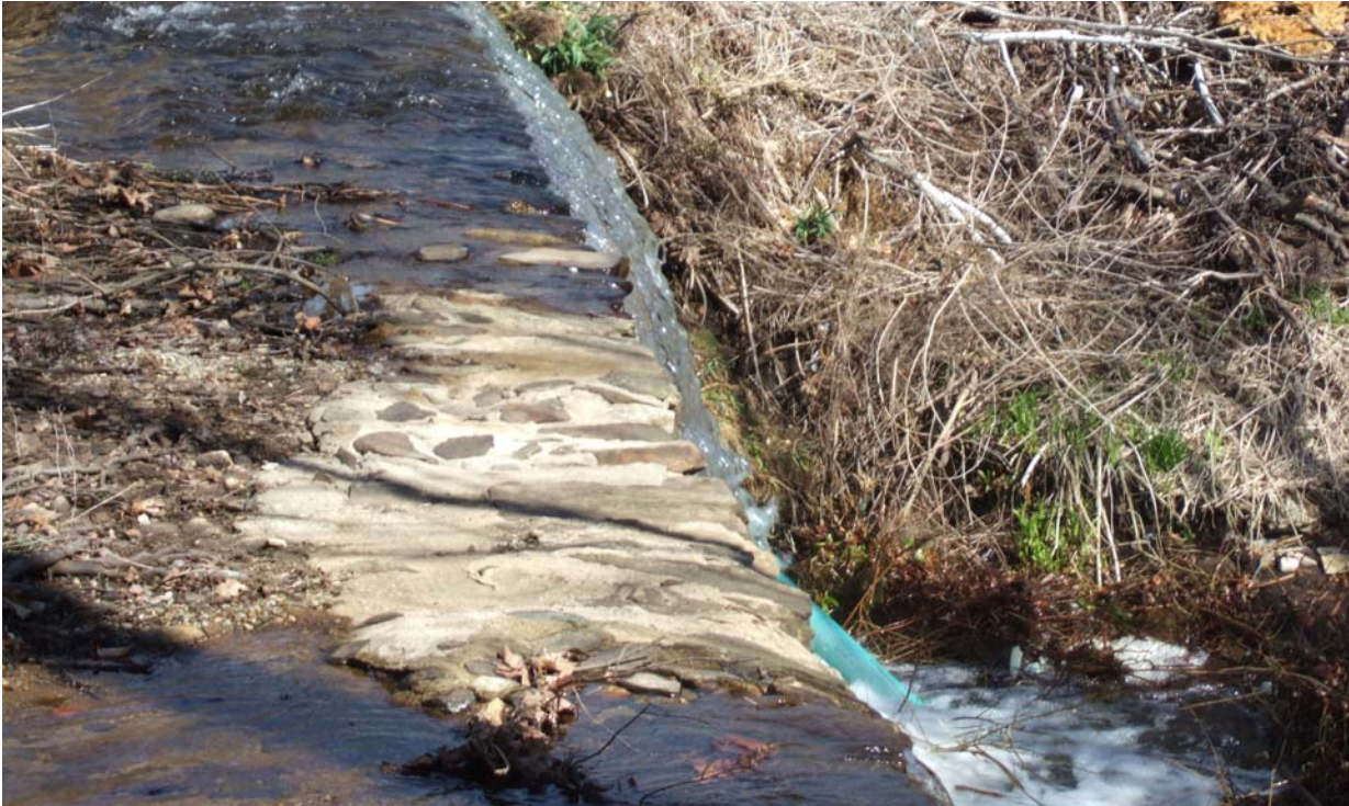
Figure 4. 3 Stone Masonry Crest of the Hughesdale Lower Pond Dam
