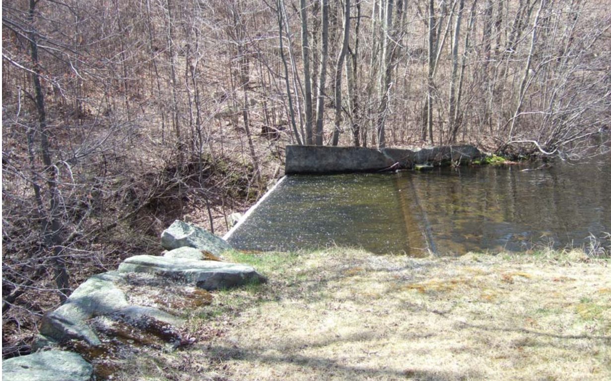
Figure 4. 6 The Hughesdale Upper Pond Dam
