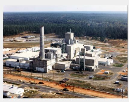
houses production facilities that include a fuel and target fabrication facility, five production reactors, two chemical separations areas, a tritium processing facility, a heavy water rework plant, a uranium fuel processing facility, and the Savannah River Technology Center (formerly Savannah River Laboratory).
