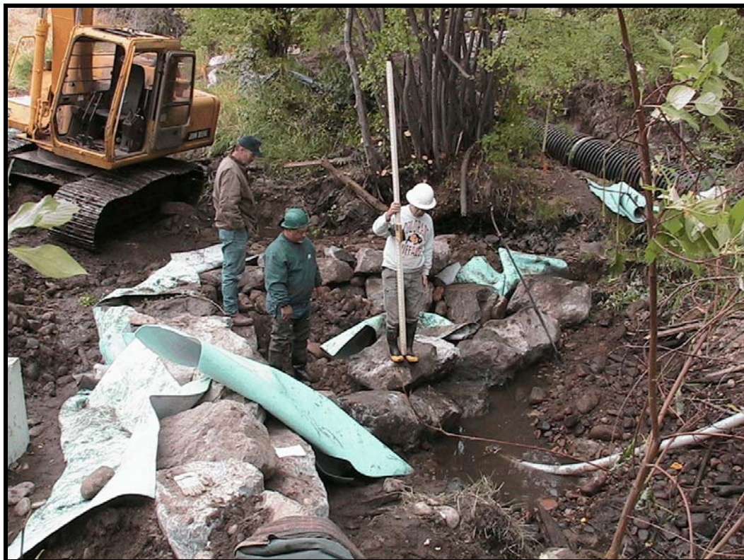
Photo A-6. Looking upstream at Weir No. 1. A section of the dewatering pipe can be seen at the upper right; the seepage-pump line is at lower right; and the new diversion box is at the lower left.
