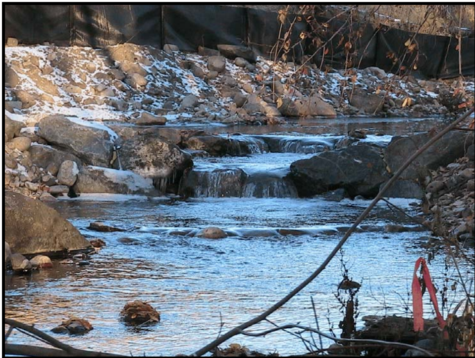
Photo A-22. A closer view of Weir No. 1 on November 15.
