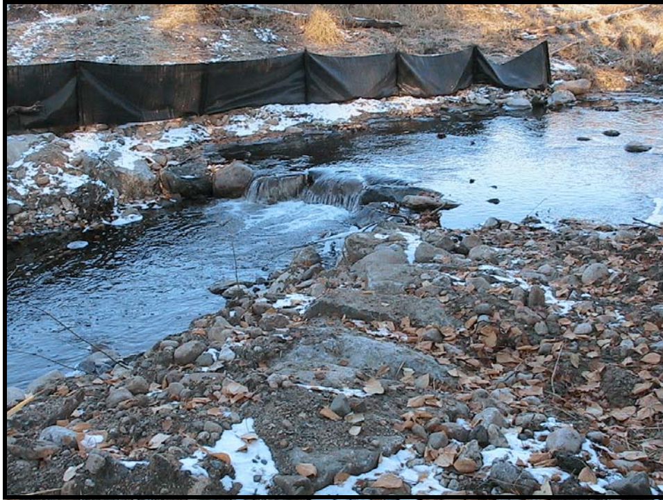
Photo A-19. Weir No. 2 during low flow on November 15, 2003. The silt fence in the background will remain in place until the spring of 2004.
