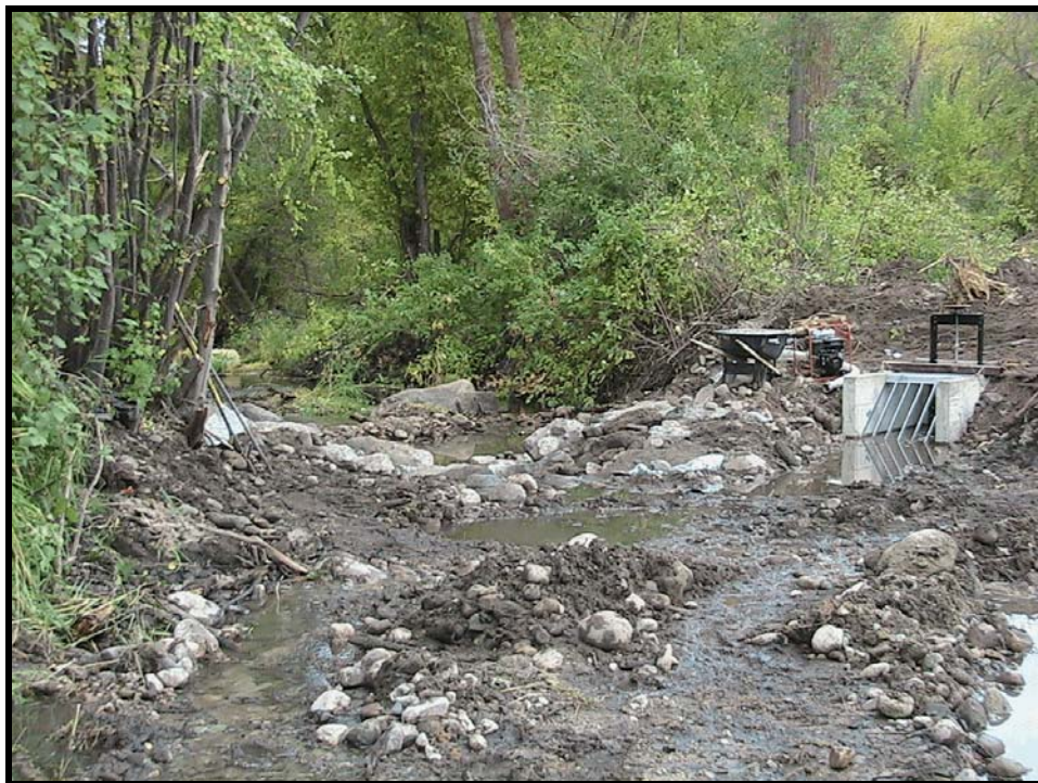
Photo A-10. Looking downstream at Weir No. 1, which has been lined with geotextile and then backfilled. The pipe trench has also been backfilled.
