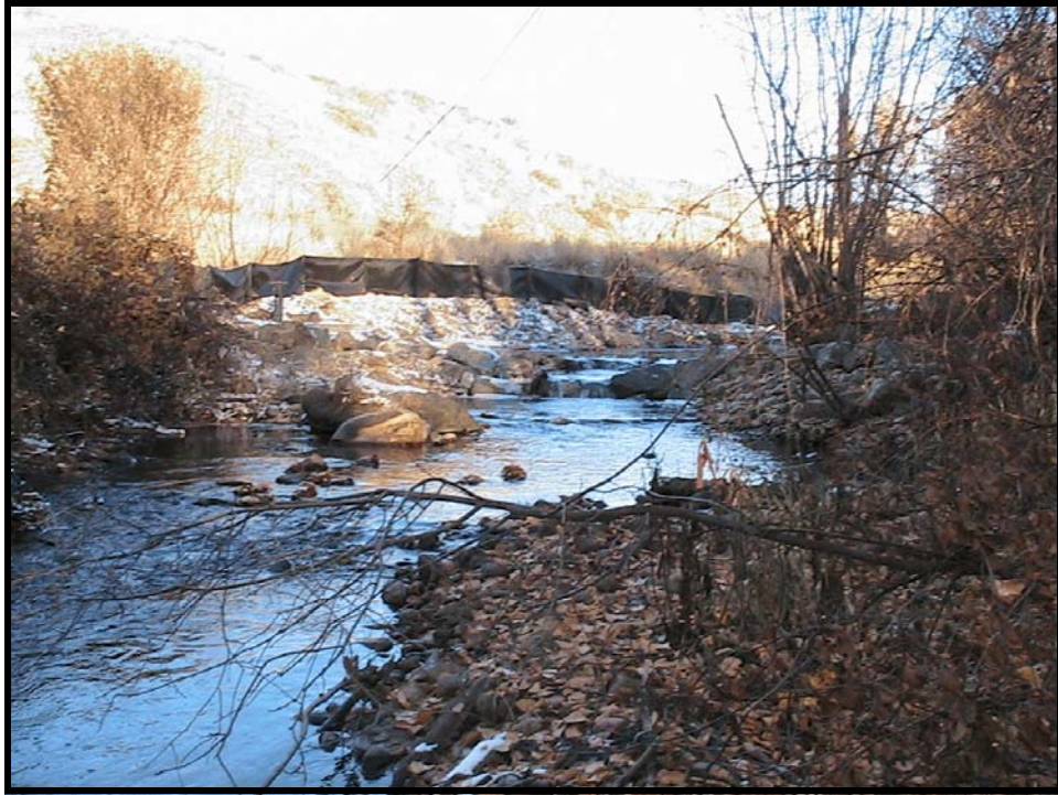
Photo A-21. Looking upstream from the exit of the fish bypass. Weir No. 1 is shown in the center of the picture.
