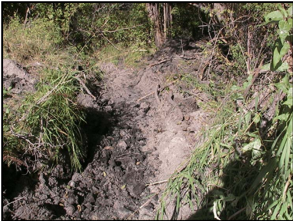
Photo A-14. Downstream of the ramp flume, more cleaned-out ditch.
