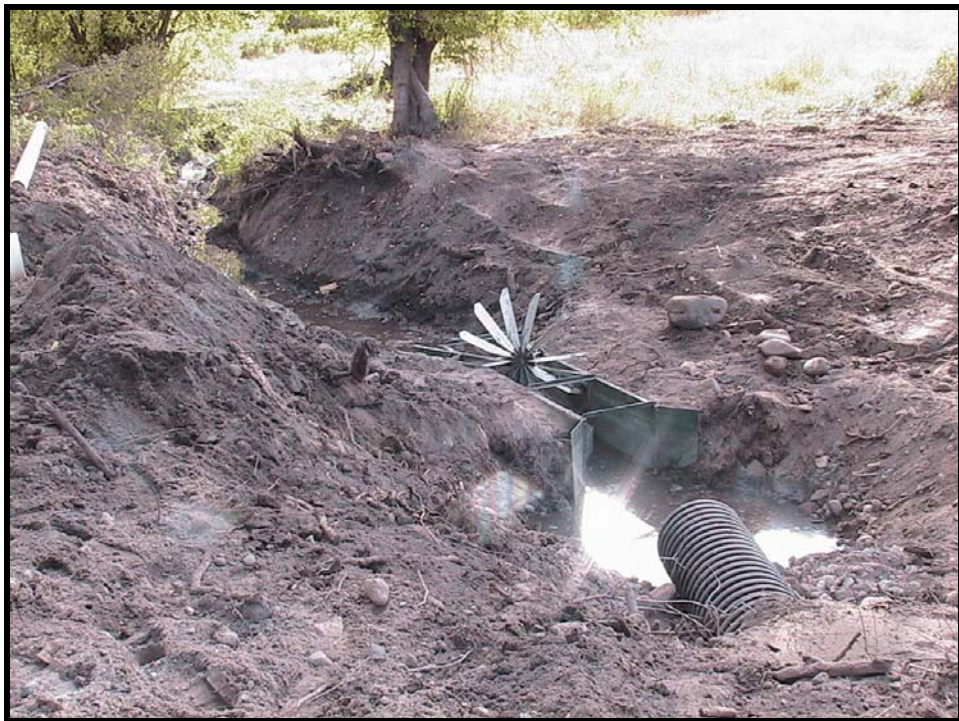
Photo A-16. The diversion pipe extension and the ditch transition at the fish screen. Note the benching of the ditch slopes.
