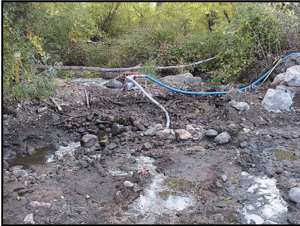
Photo A-3. Looking downstream at the double-drop Weir No. 1; rock has been placed and tied into the right bank. This is the upper portion of the A-shaped weir. The suction pump in center picture is sending seepage water into the woods.
