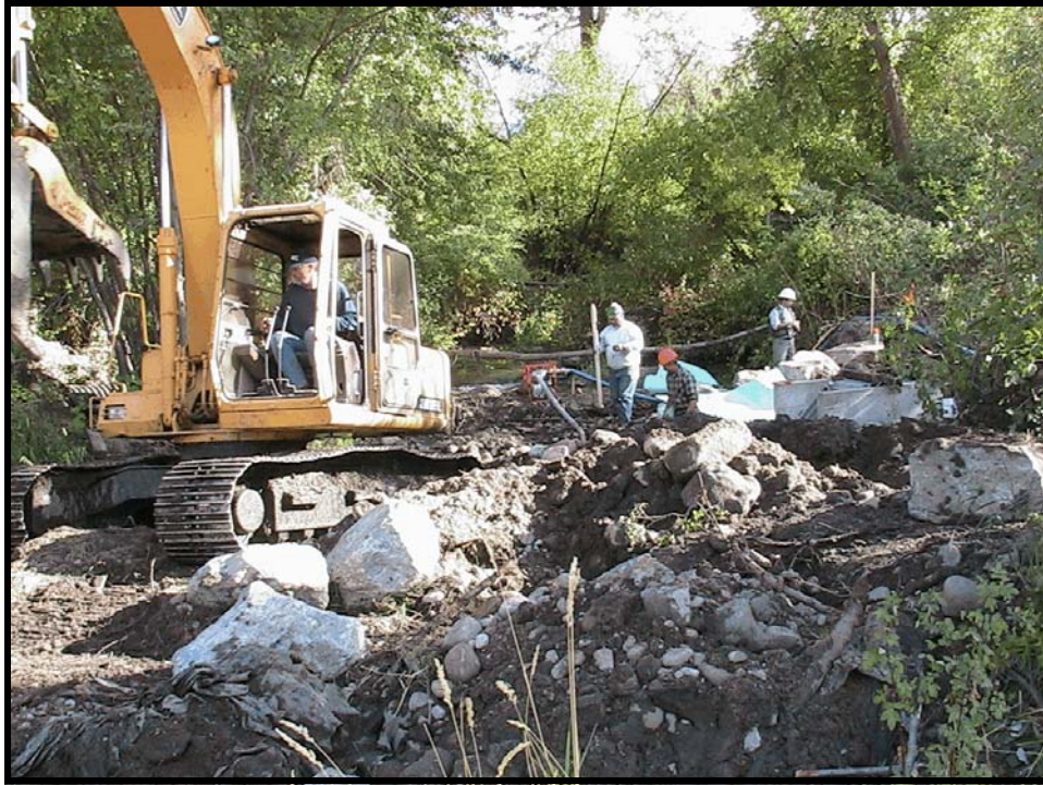
Photo A-9. Looking downstream, the new diversion structure (at middle right) has been set.
