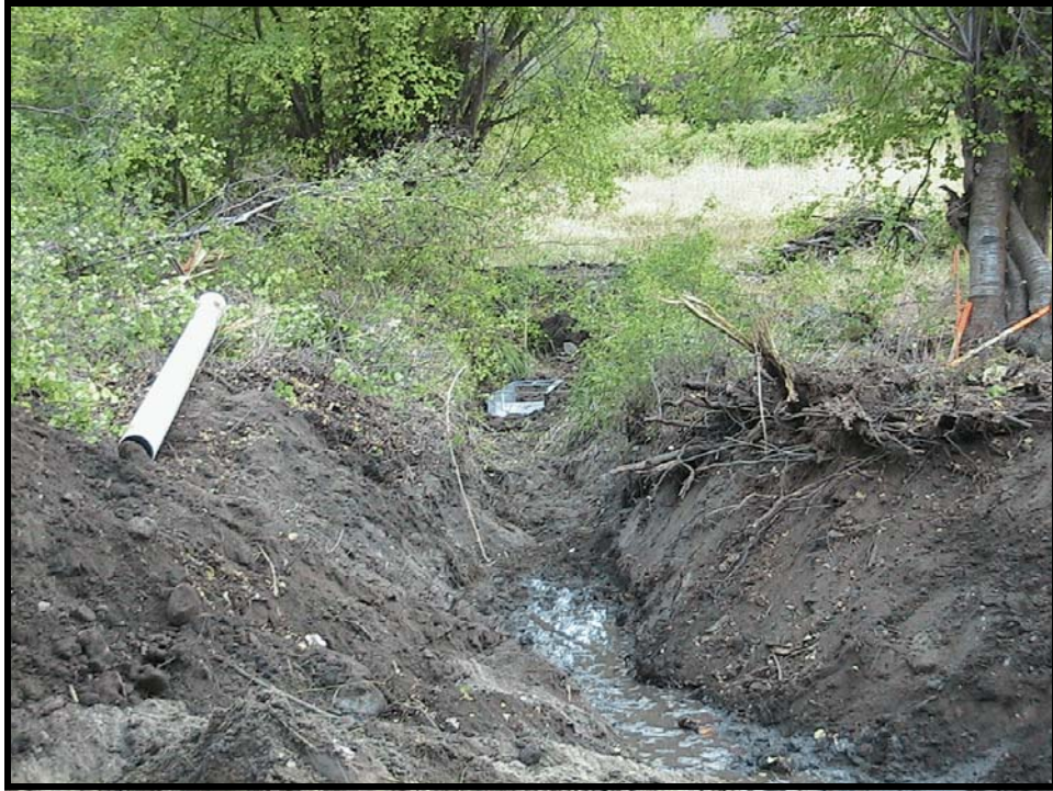
Photo A-13. Along the diversion ditch, just downstream from the fish screen. The new ramp flume is shown near the center of the picture. This portion of the ditch have been cleared of vegetation and deepened.
