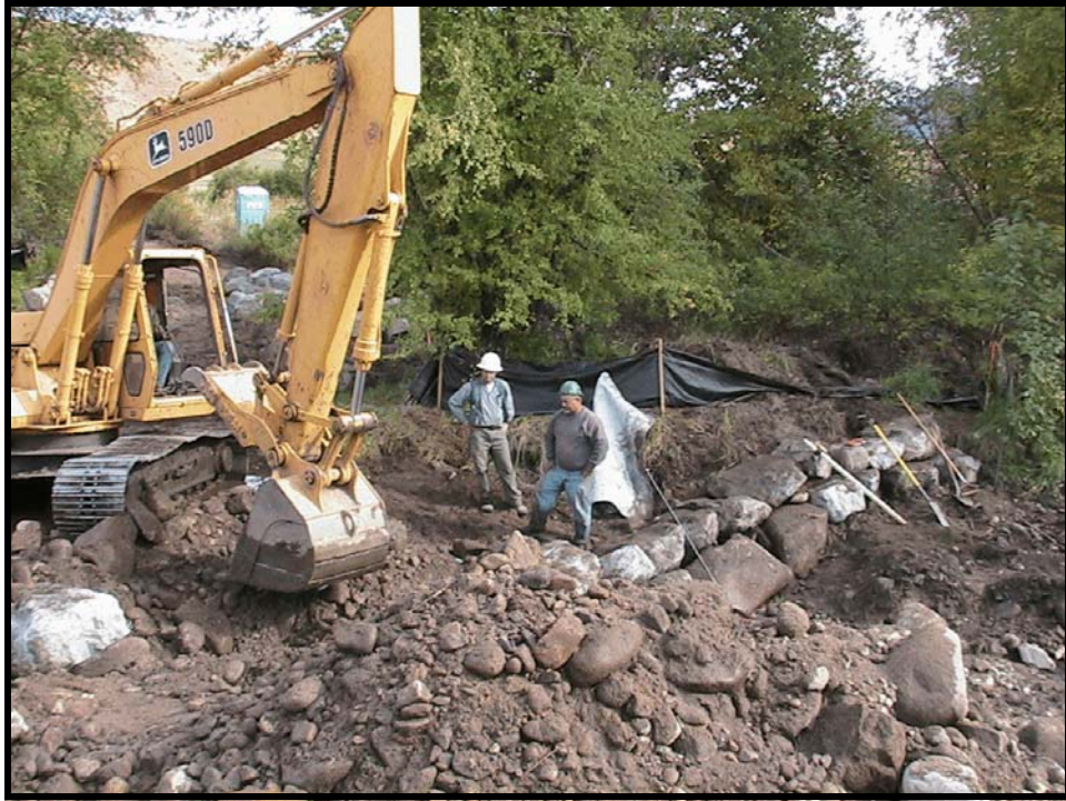
Photo A-17. Looking across Beaver Creek to the left arm of Weir No. 2.
