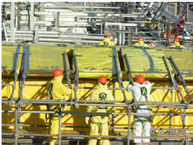
Exhibit 4-25: Jumpers prior to removal
