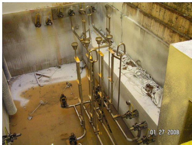
Exhibit 4-27: New jumpers installed
