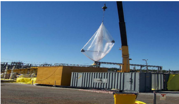
Exhibit 4-21: Sleeved jumper lifted out of the pit.
