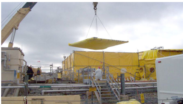
Exhibit 4-17: Removable roofs to allow access.
