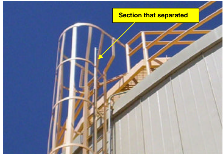
Figure 1. Rail Installation at RTC
