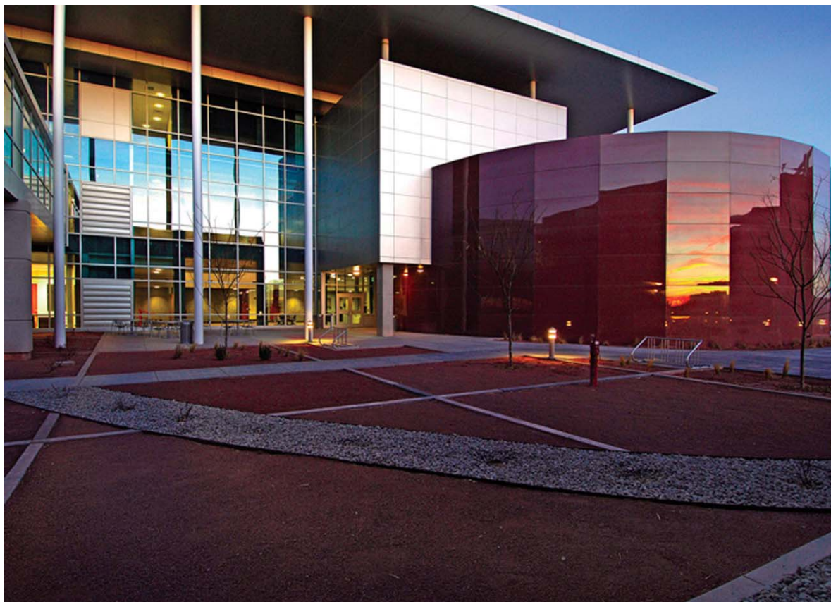
MESA: The setting sun reflects off the glass of the cylindrical training center attached to Sandia's new MicroLab building. The building is the second of three to come online of the defense laboratory's $500 million MESA project.
